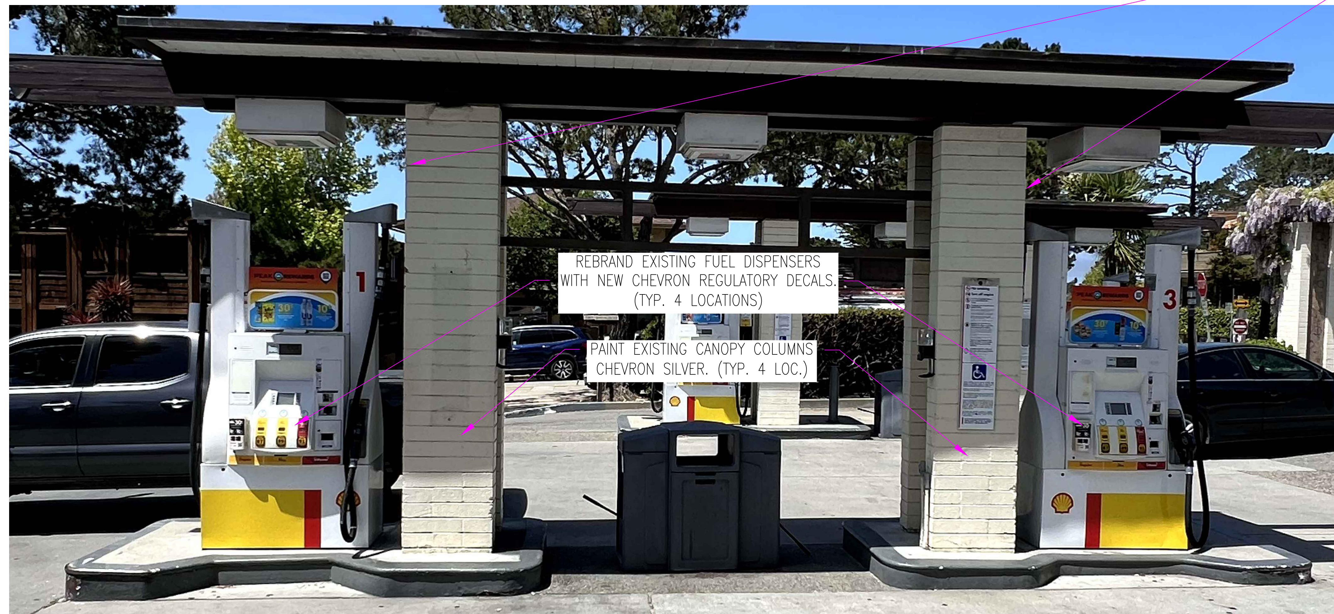
EXISTING SHELL FUEL DISPENSERS
