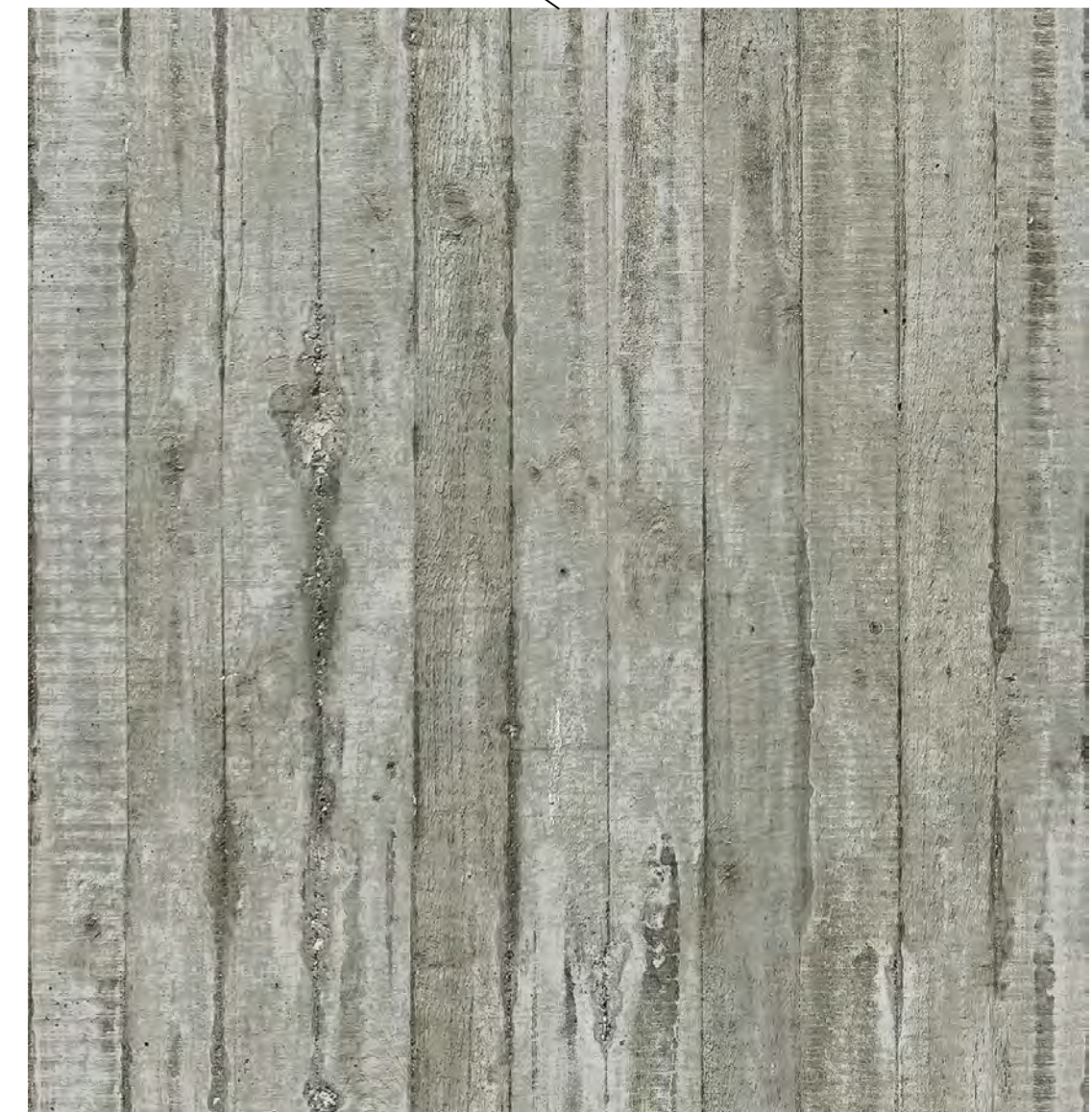
EXTERIOR SIDING VERTICAL BOARD FORM CONCRETE
