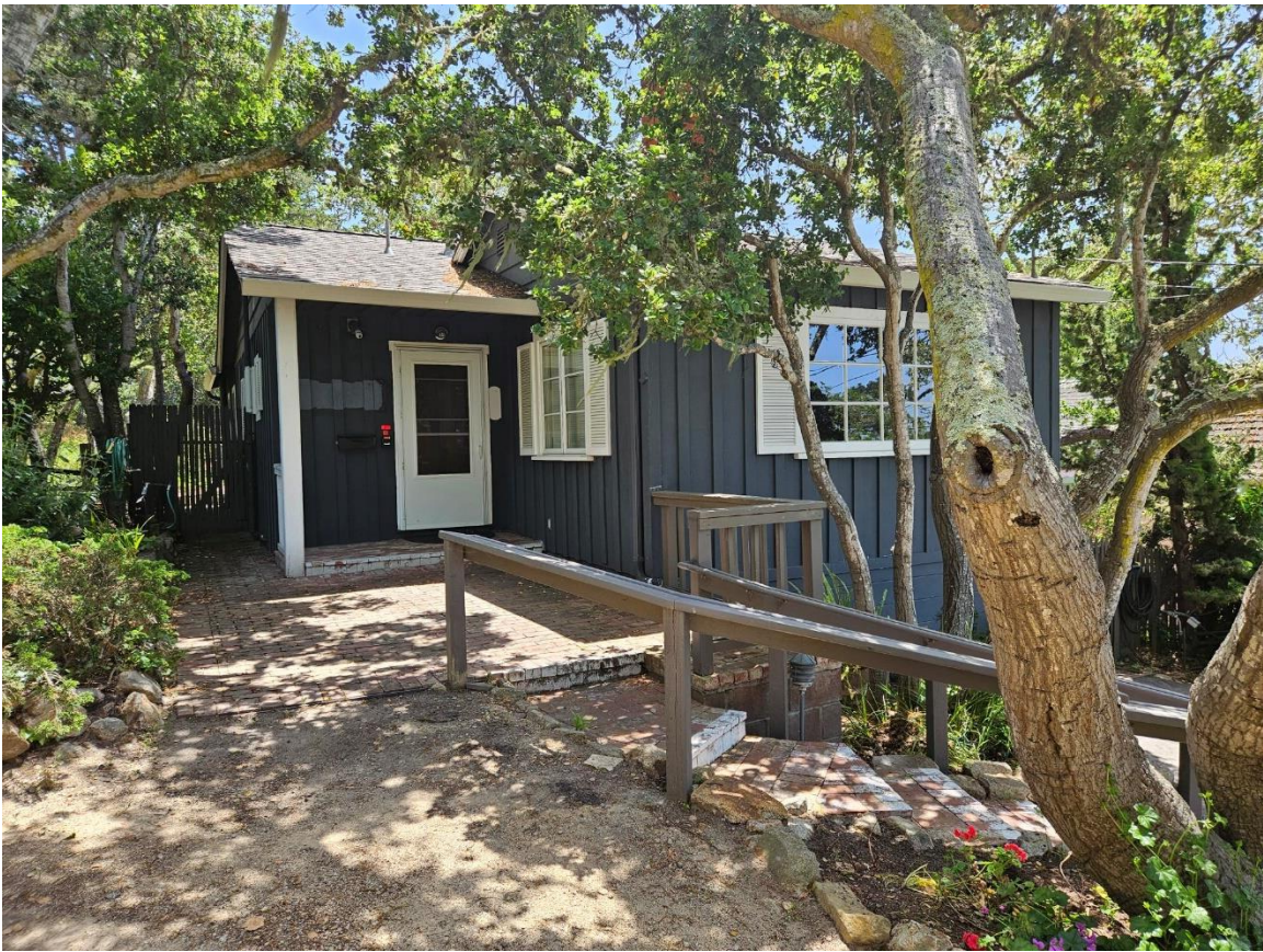
View of front elevation looking southeast.
