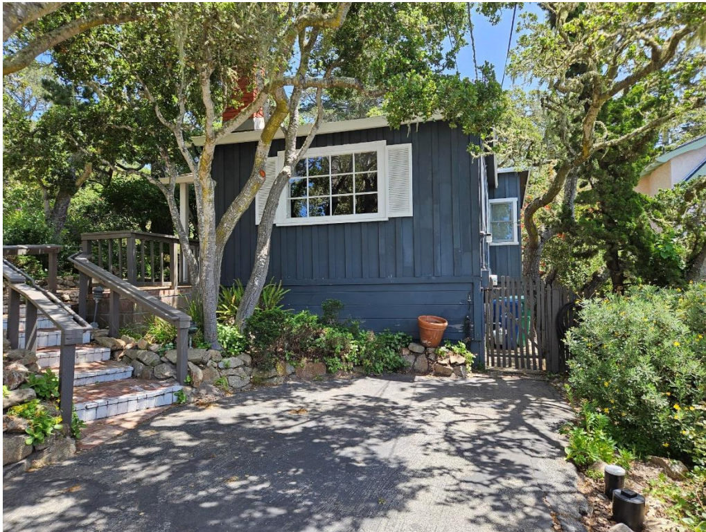
View of front elevation looking northeast.
