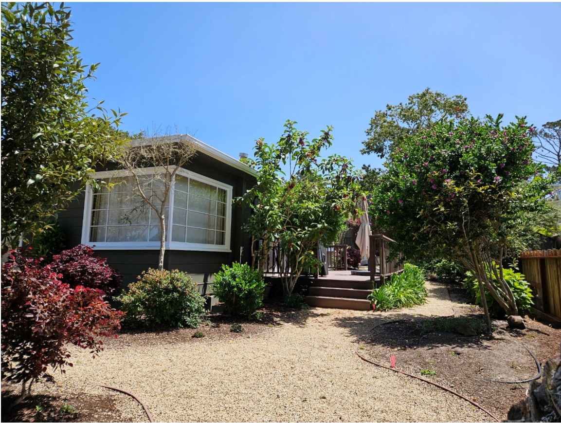
View of south elevation.
