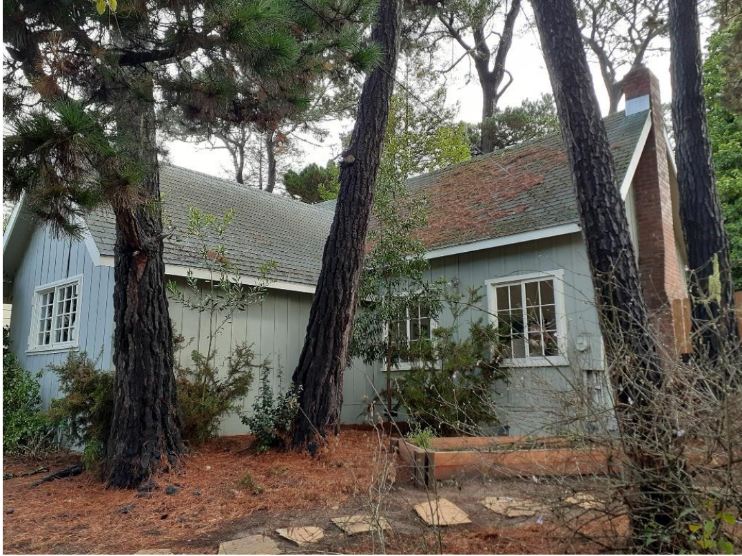
View of house looking northeast
