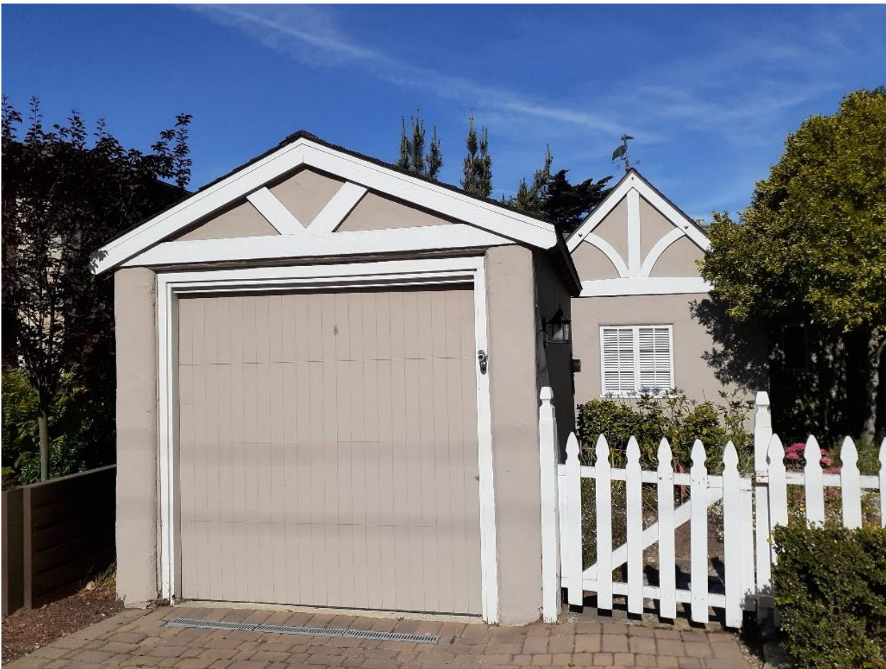
E.P. Young Spec House Garage (original double doors were replaced in 1998)
