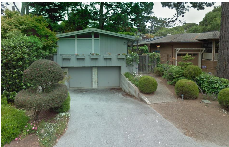
11. 2011 Photograph of the Residence:
