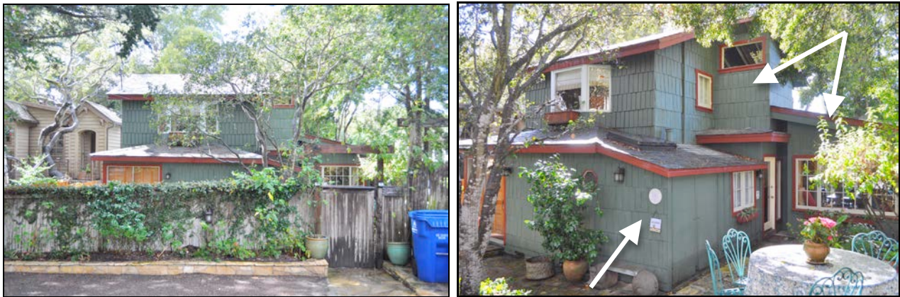
Figures 1 and 2. Left image shows the east (Santa Fe St.) elevation. Right image details the east and north elevations. The stairwell and shed-roofed dining room additions (arrows) were installed in 1983. The bathroom addition to the first floor (arrow) was installed in 1993.
