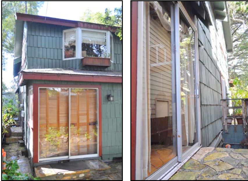
Figures 3 and 4. Left image details the east elevation, southeast corner, showing sliding glass doors and upper-floor bay window added in the 1990s. Right image looks east along the south elevation, showing sliding glass doors added in the 1960s. The original dining room was removed in 1983.
