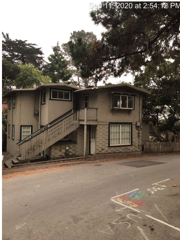
North (3 rd Avenue)
