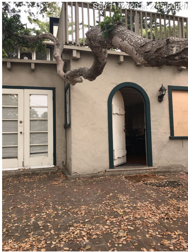
West Elevation (Roof Deck above)
