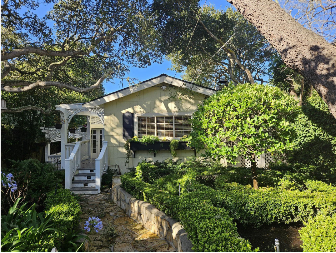
Figure 2: View of front elevation.
