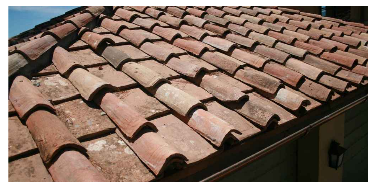
O - ROMAN STYLE CAP & PAN CLAY TILE ROOF, BUILDING-2 & NORTH WING OF BUILDING-1
