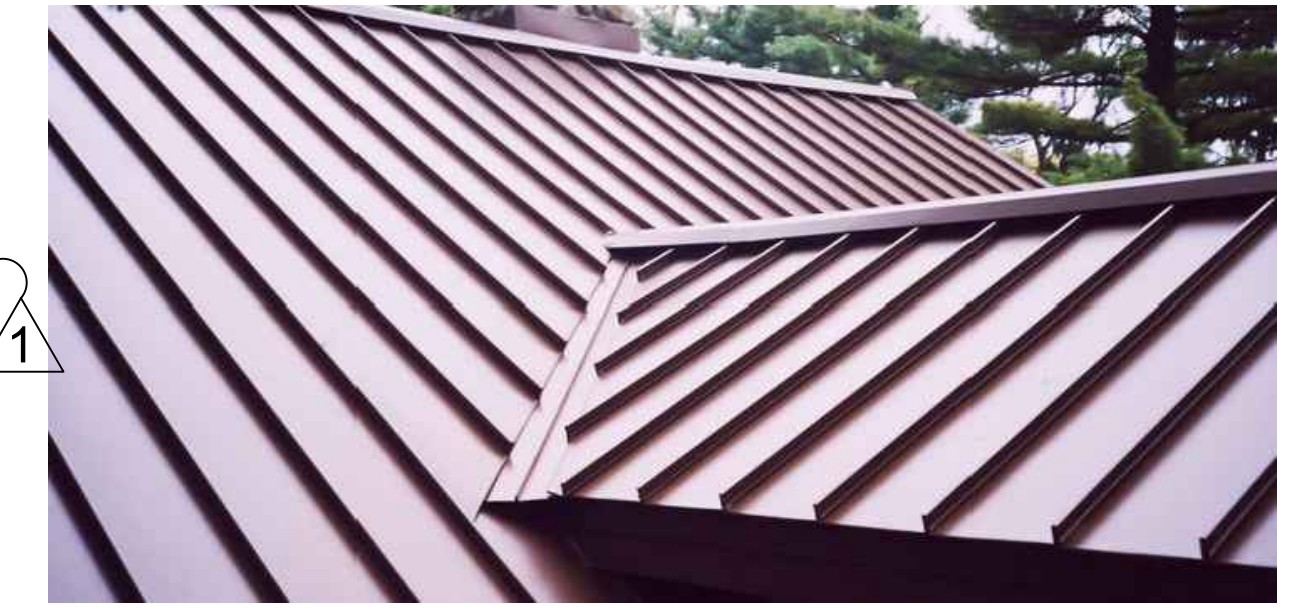
STANDING SEAM METAL ROOFING
