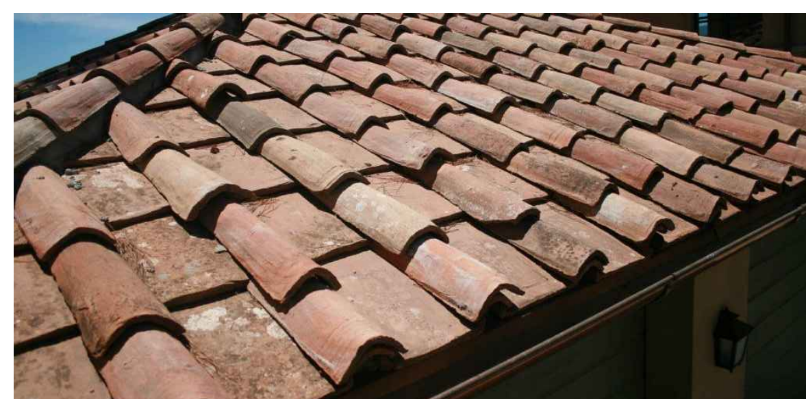
O - ROMAN STYLE CAP & PAN CLAY TILE ROOF, BUILDING-2
