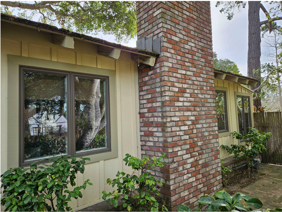
Figure 3: View of west elevation.
