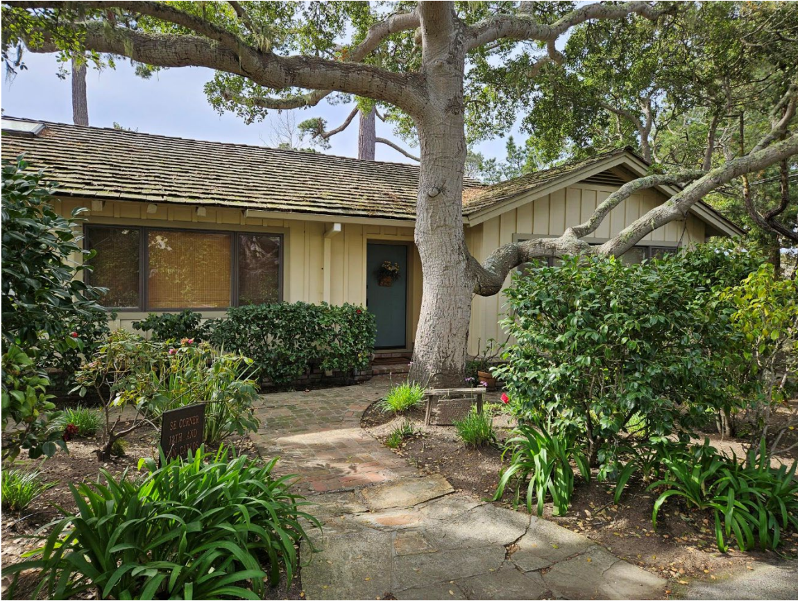
Figure 2: View of front elevation.
