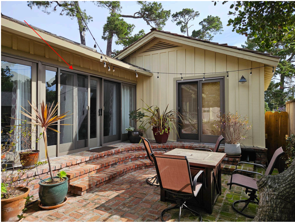
Figure 5: View of solarium, rear elevation.
