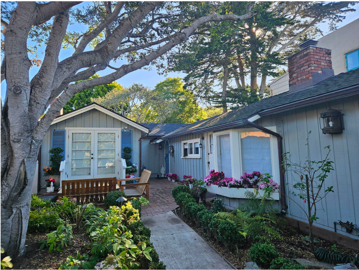
Figure 1: View of front elevation looking east from Carmelo Street.
