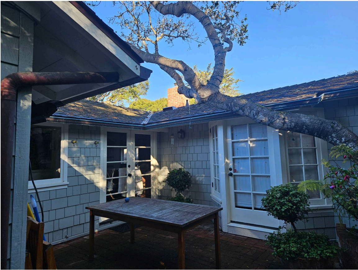
Figure 2: View of rear elevation.
