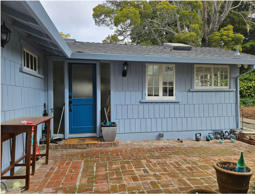
Figure 3: View of front door alteration.
