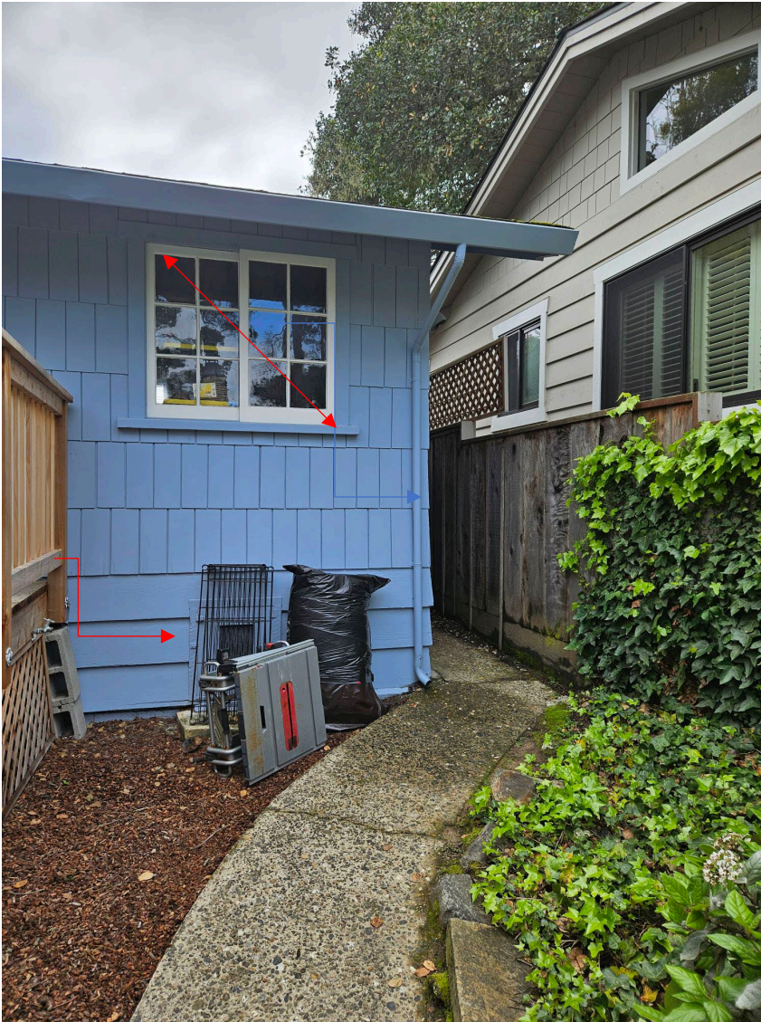
Figure 5: View of Murphy features: extended lintels, sills, and horizontal siding at basement level.
