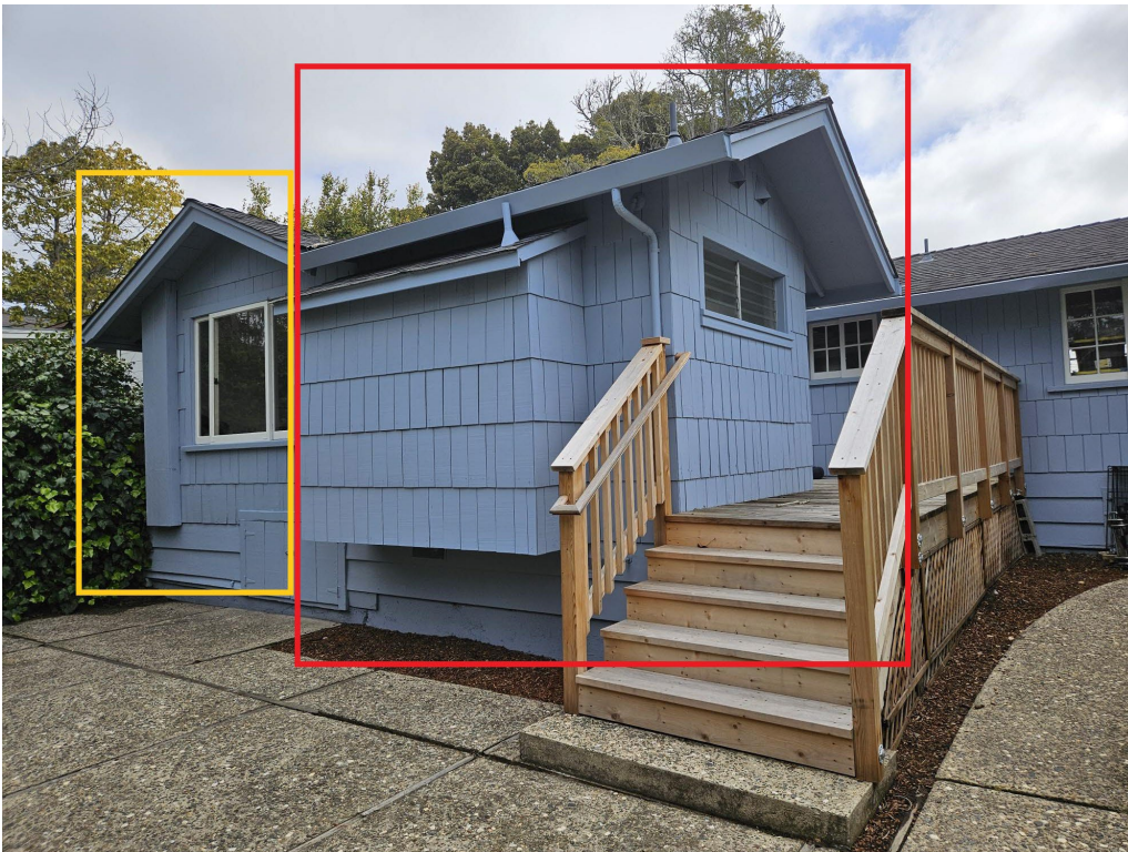
Figure 4: Rear Elevation. 1964 addition is outlined in red; 1929 addition is outlined in yellow.
