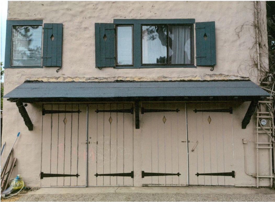
Figure 4: View of original garage doors and shutters, 2017.
