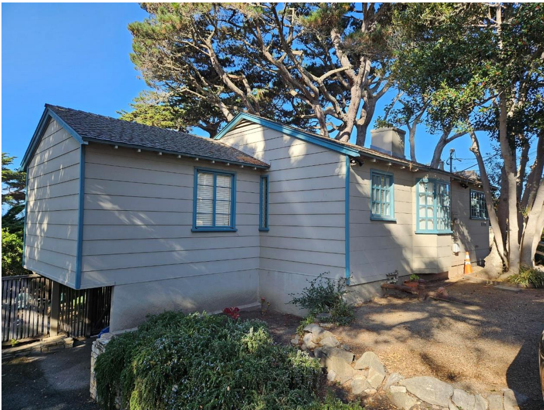
View of residence looking northwest from San Antonio St.
