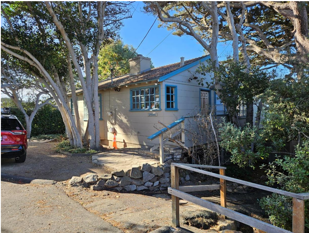
View of front elevation looking southwest.
