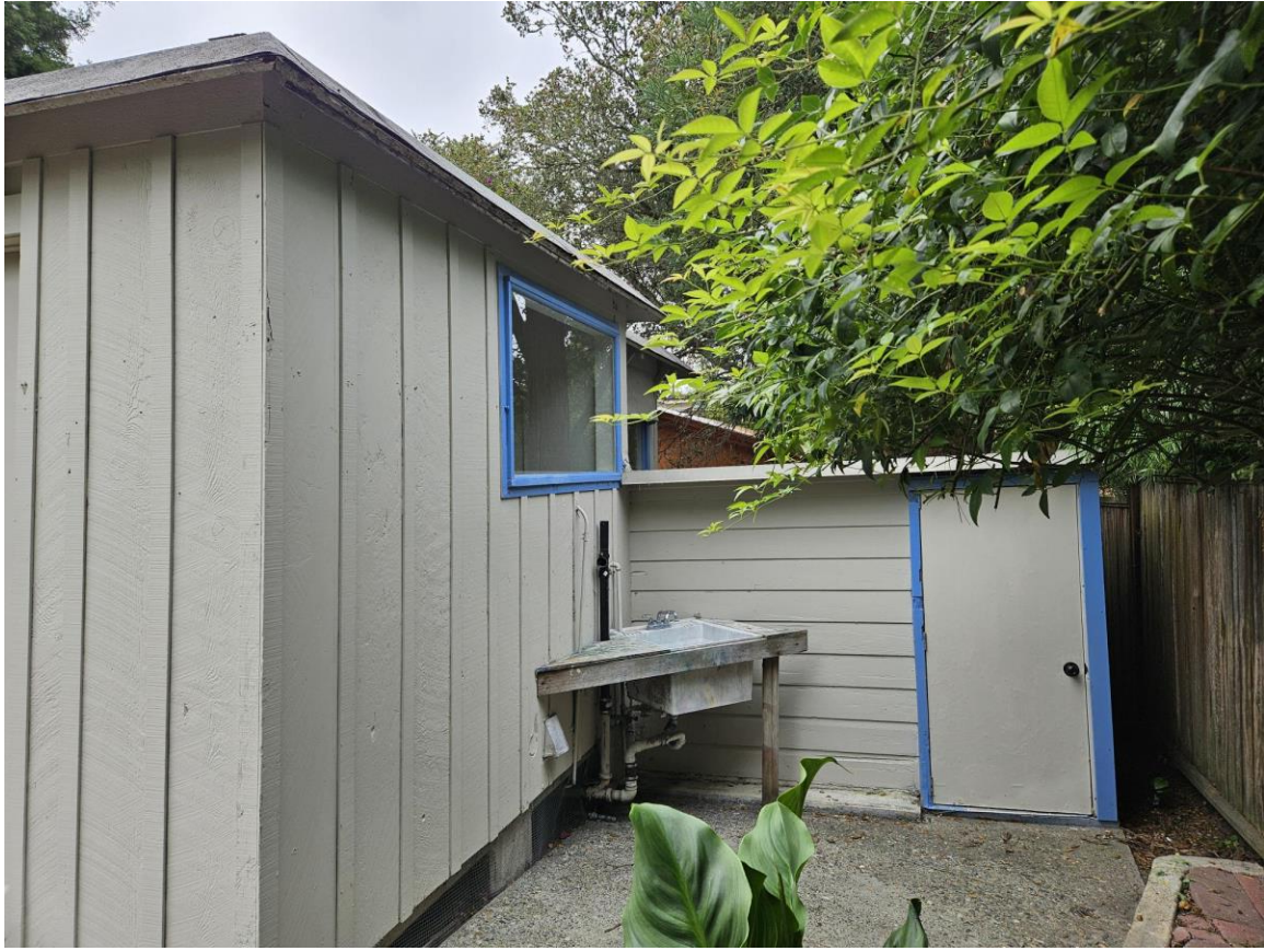
View of rear elevation.
