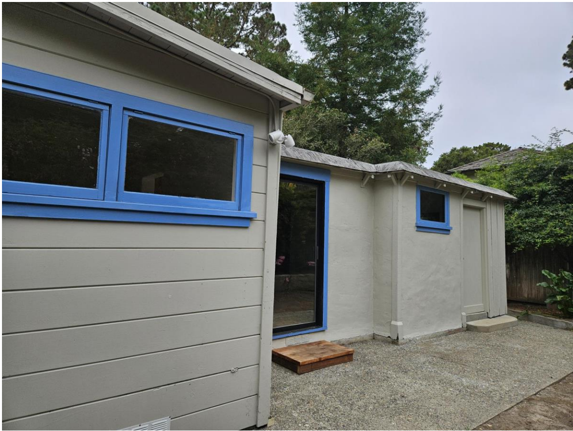
View of north elevation.
