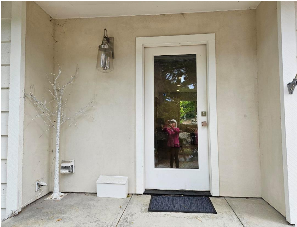
View of front entrance after 2013 remodel.
