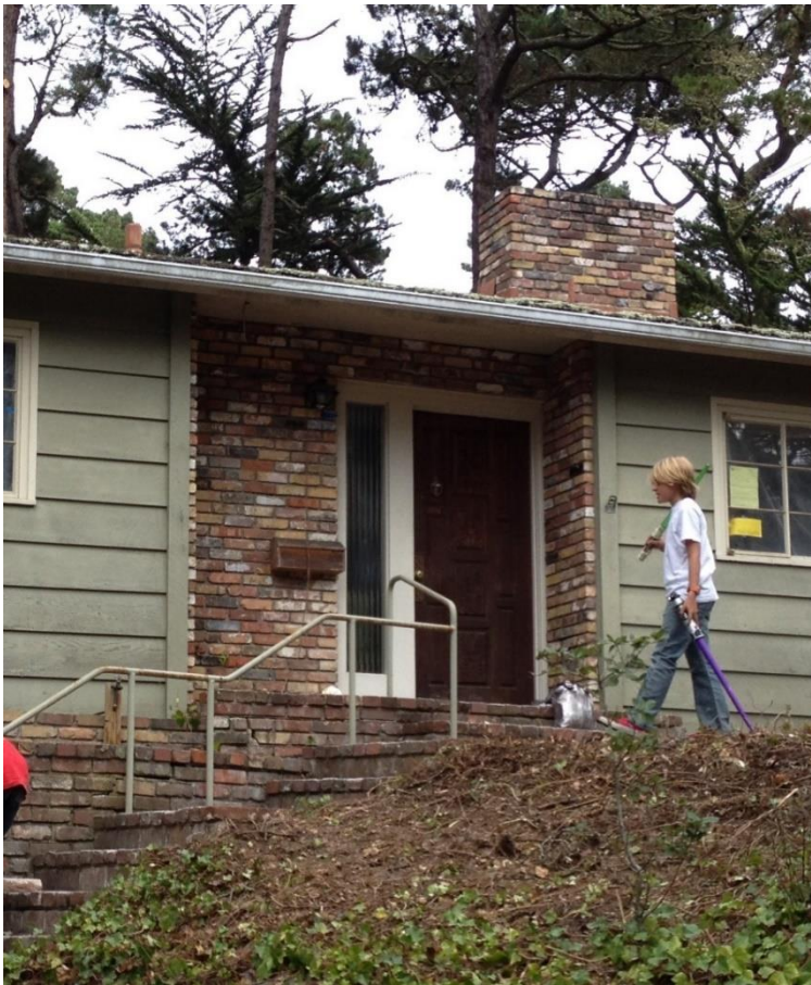
View of brick entry and chimney prior to 2013 remodel.
