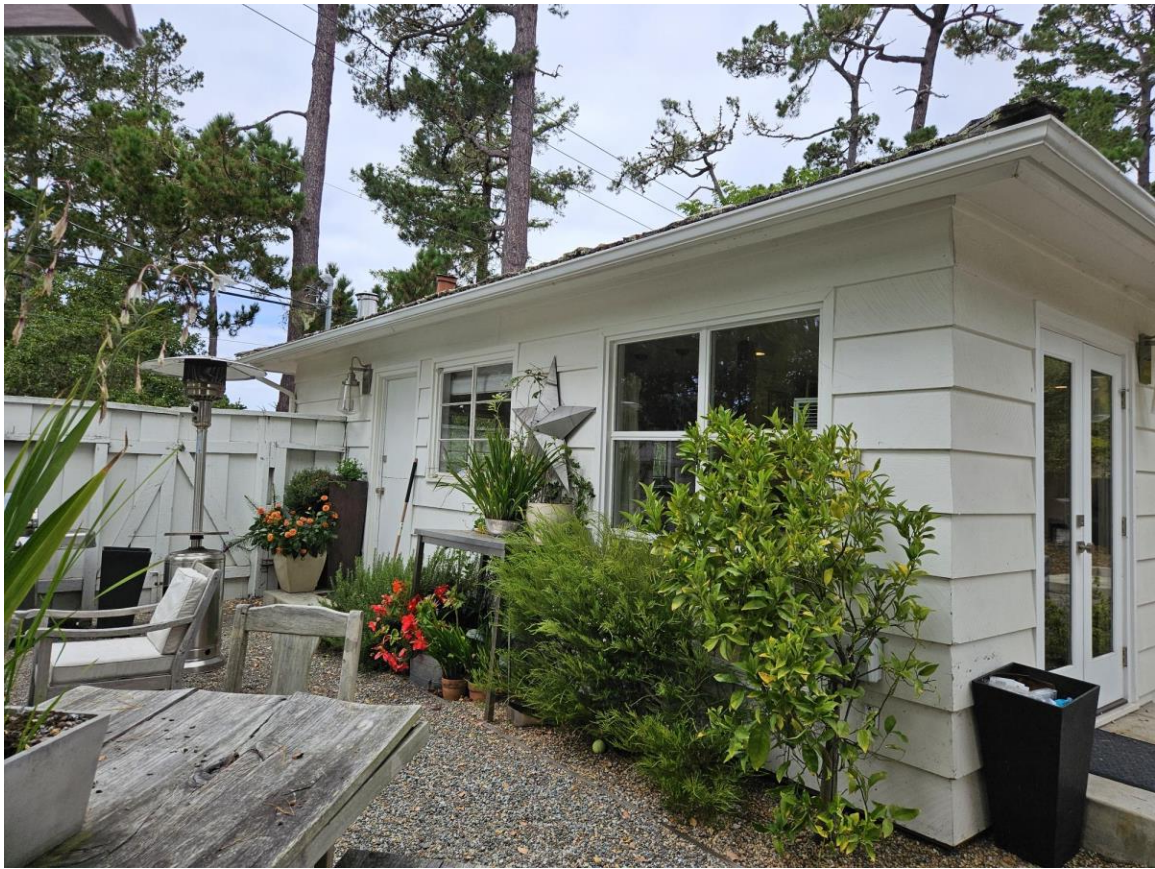
View of south elevation.
