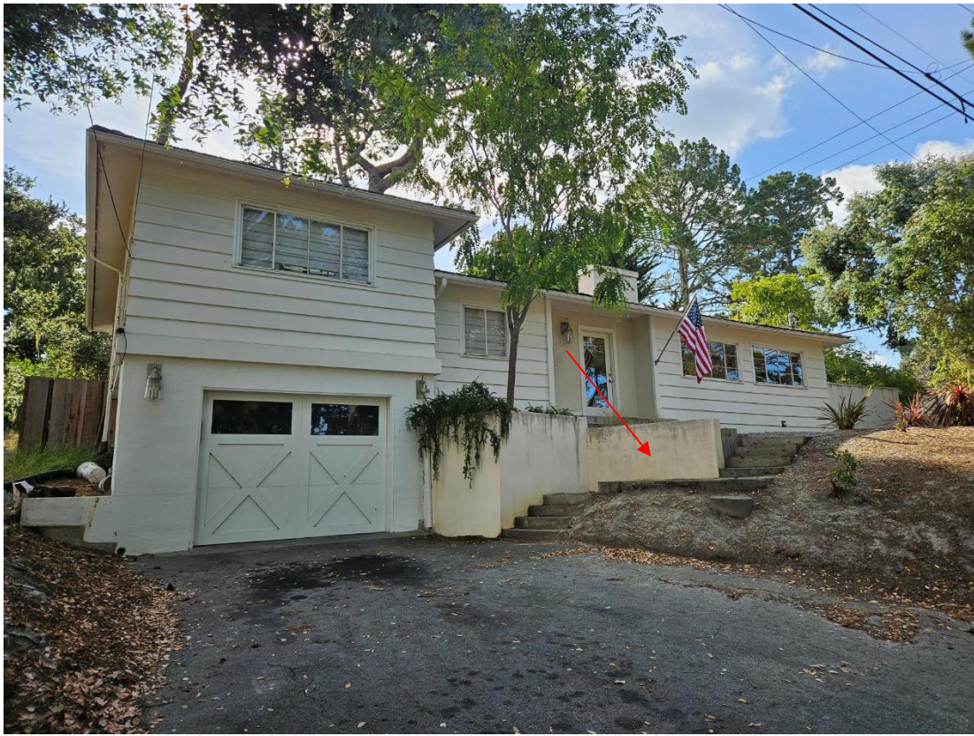
View of front elevation looking southeast. Arrow indicates new retaining wall.
