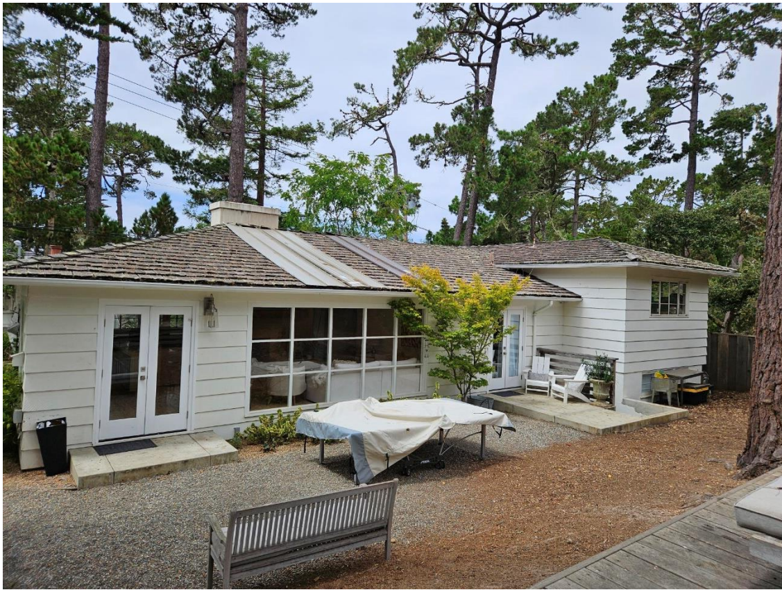
View of rear elevation.
