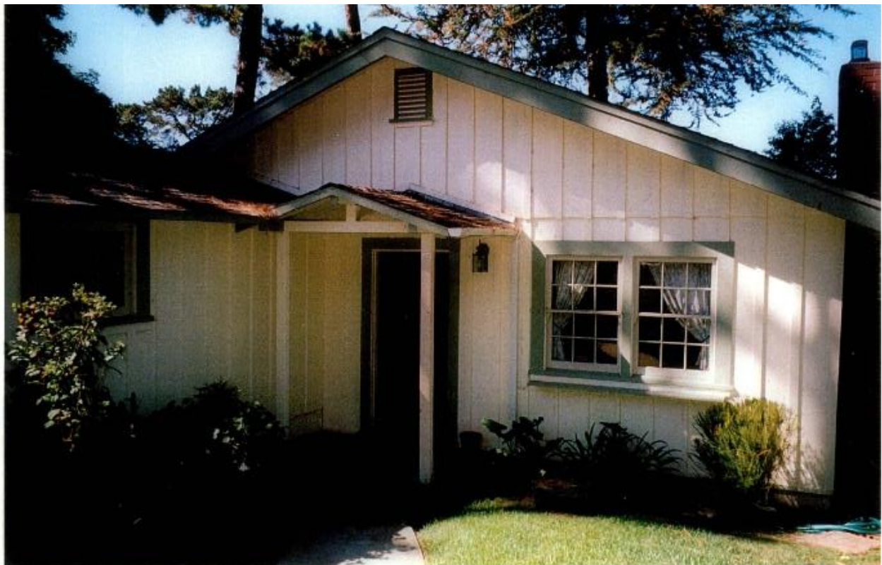
View of the front elevation, prior to 2003 remodel.
