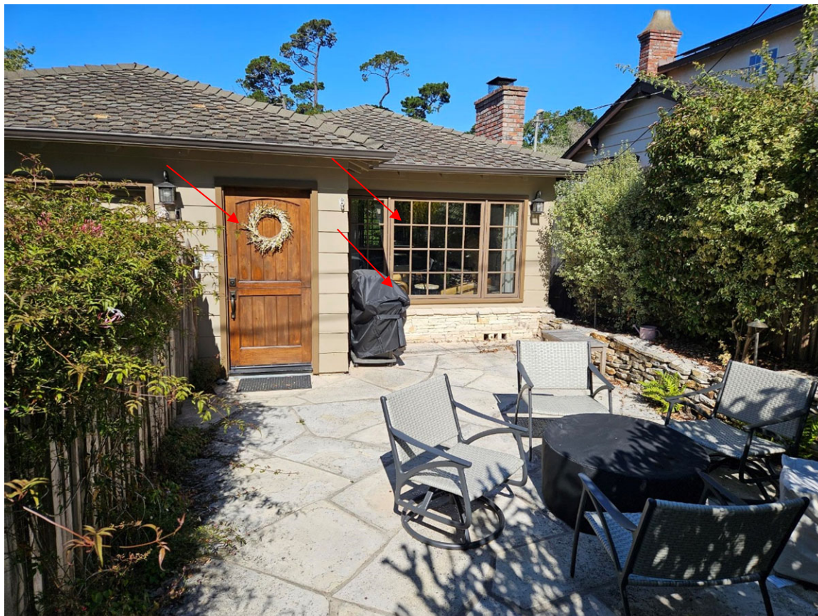
Figure 2: View of new front door and window and Carmel stone veneer.
