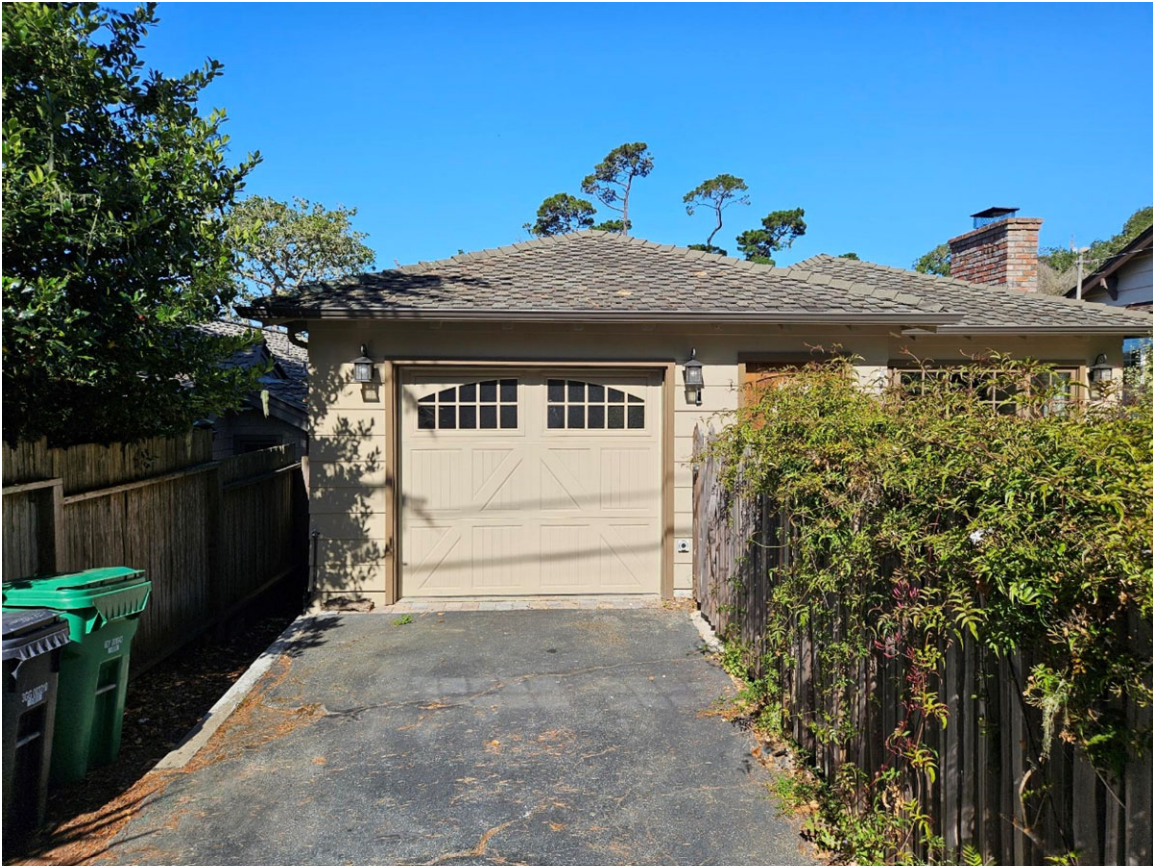
Figure 3: View of enclosed garage and new hipped roof.
