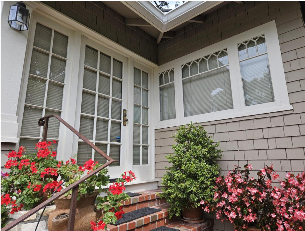
Figure 8: View of front door.
