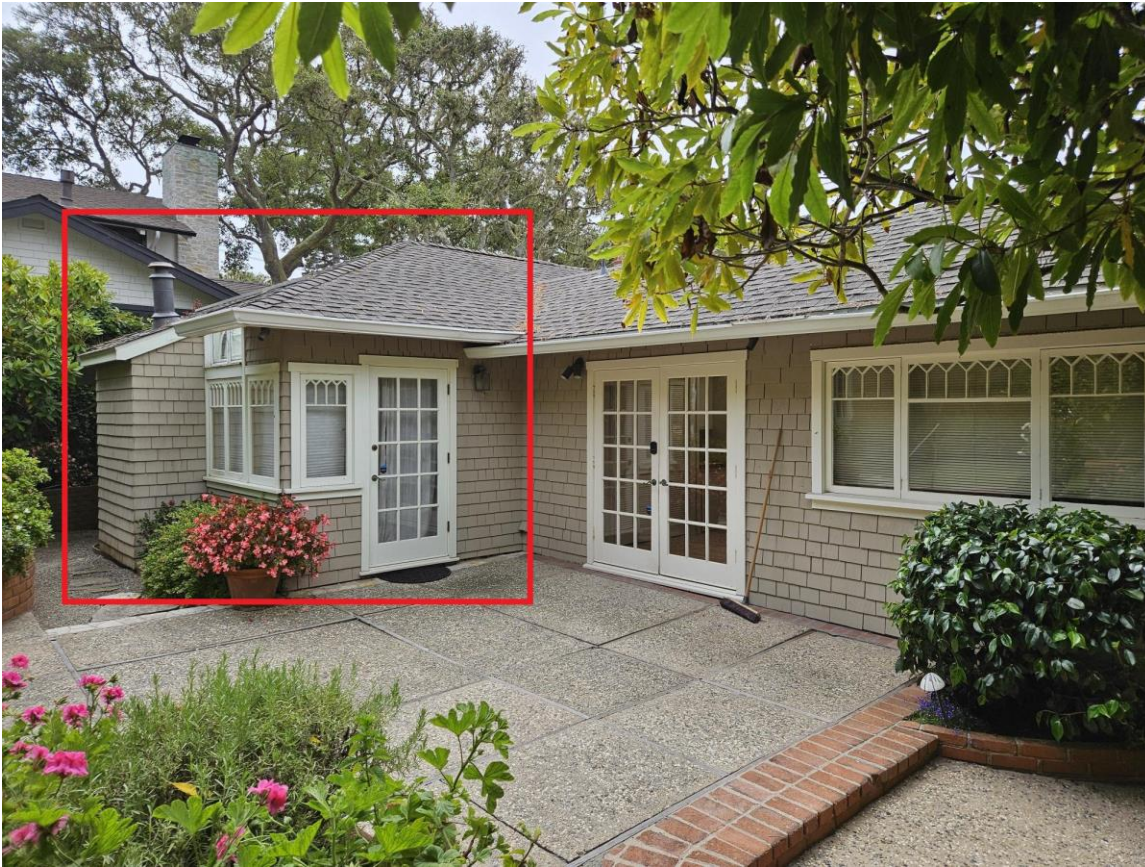
Figure 6: View of 1998 addition. All windows in this photo were moved from other locations in the house.
