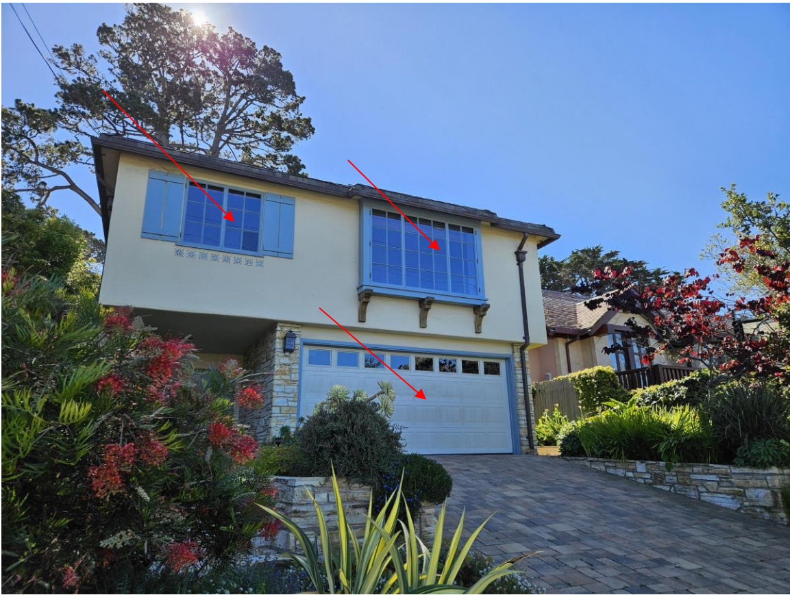
View looking southeast with new shutters, windows, inset tiles, window brackets, garage door, and stucco siding.
