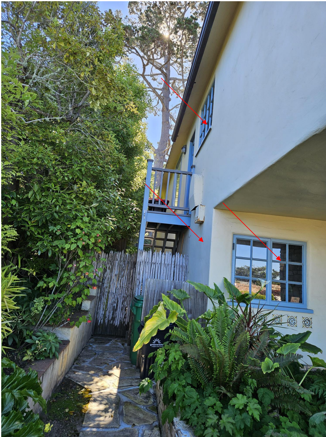
View of north elevation with stucco replacing the original stone veneer, and multi-paned window replacing the floor to ceiling fluted glass side lite.
