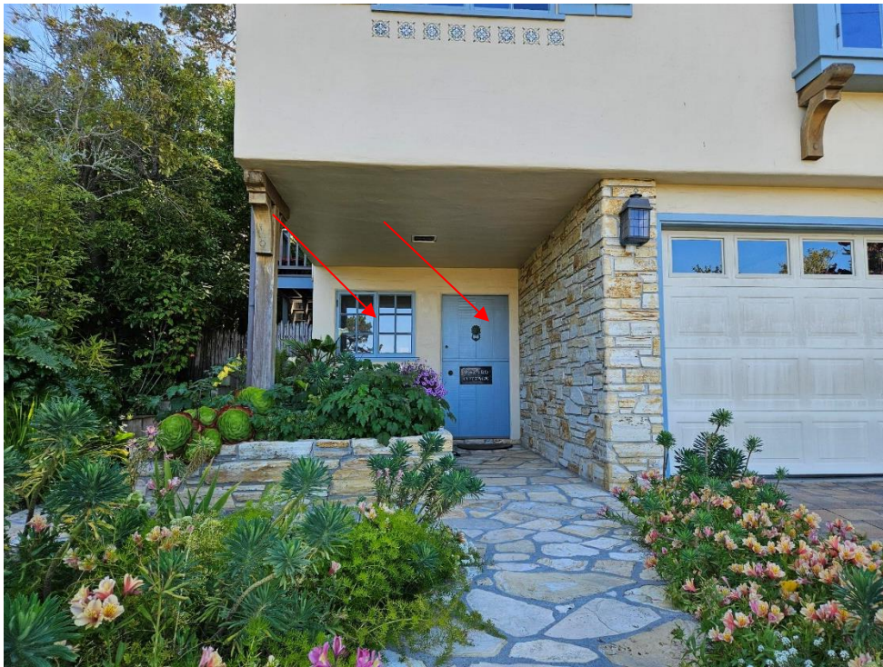
View of new Dutch door entrance and replacement window.
