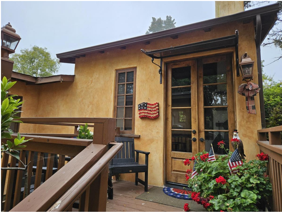
View of front deck.
