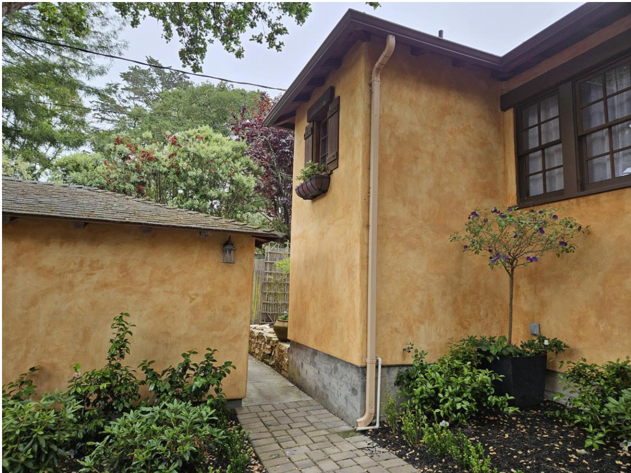
View of front addition looking north.
