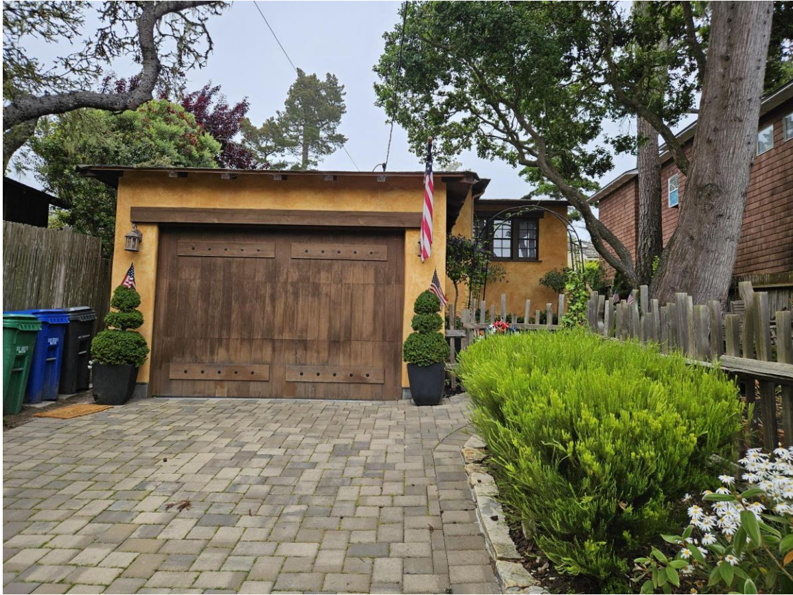
View of garage from Carpenter.
