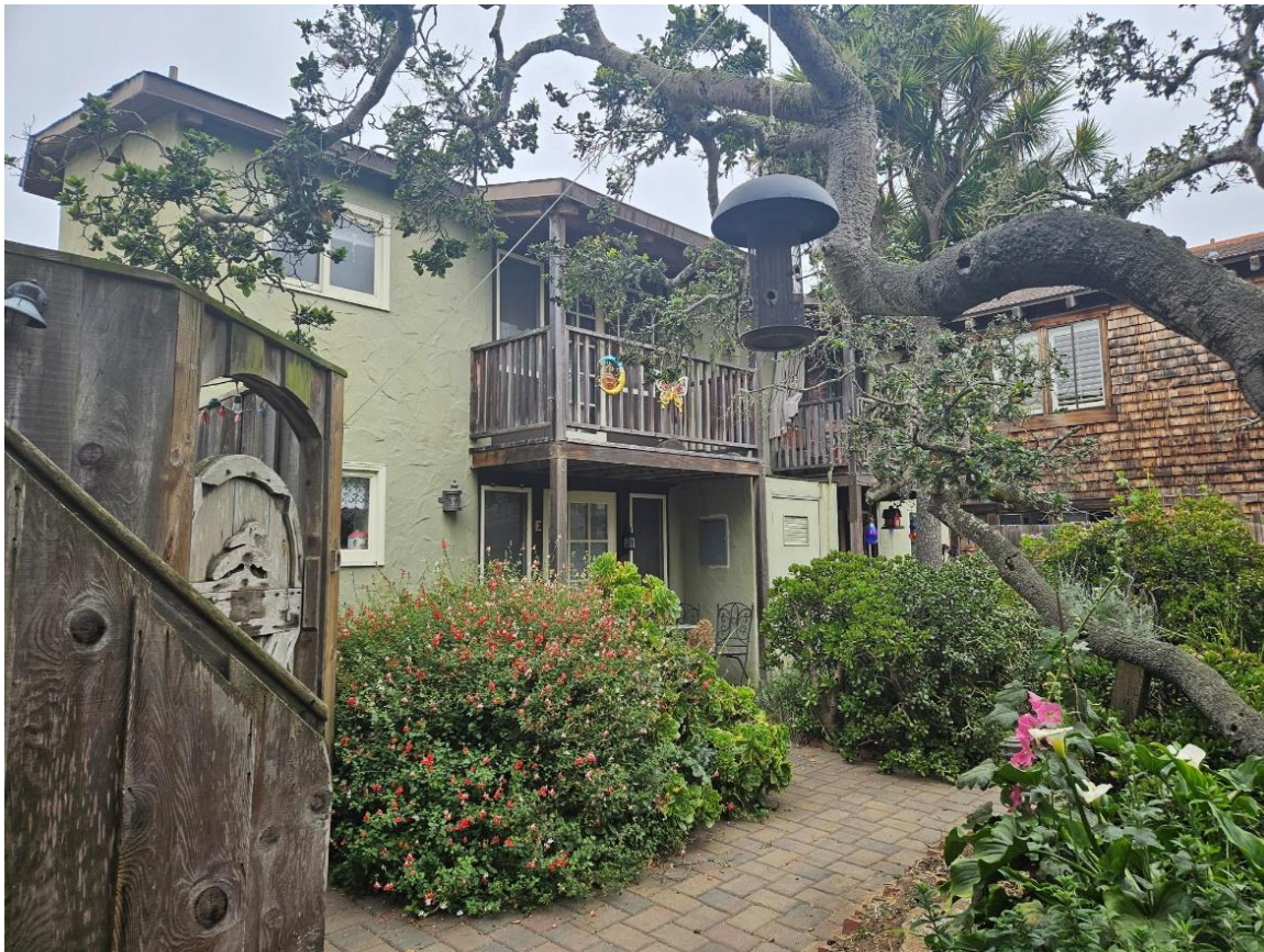
View of courtyard apartment building, west lot line.
