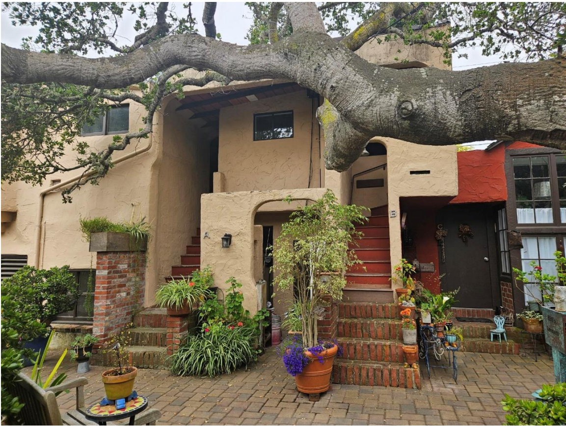
View of courtyard looking south.
