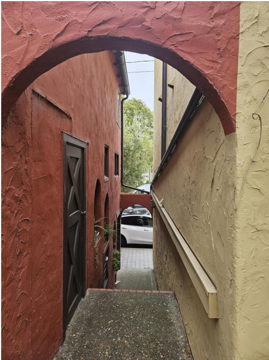
Stairs to 8 th Avenue from courtyard.
