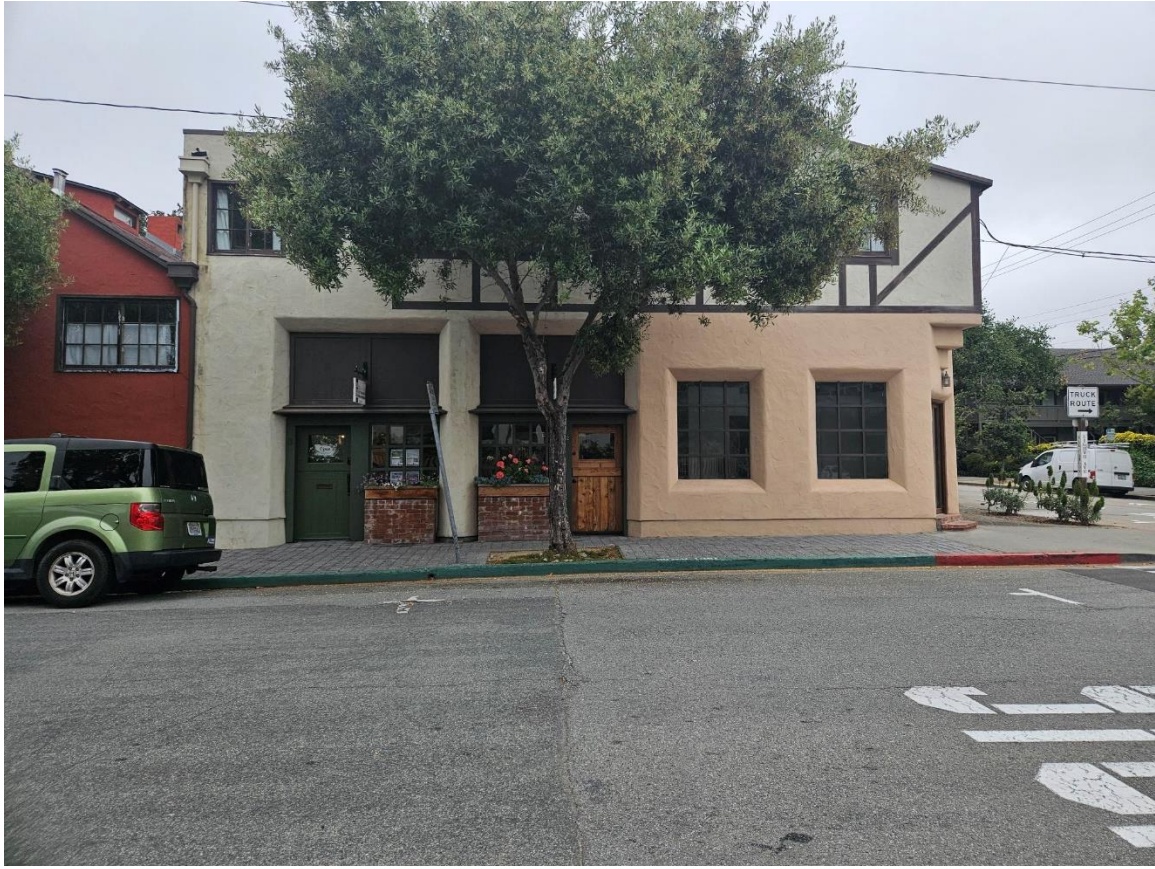
South elevation looking north.
