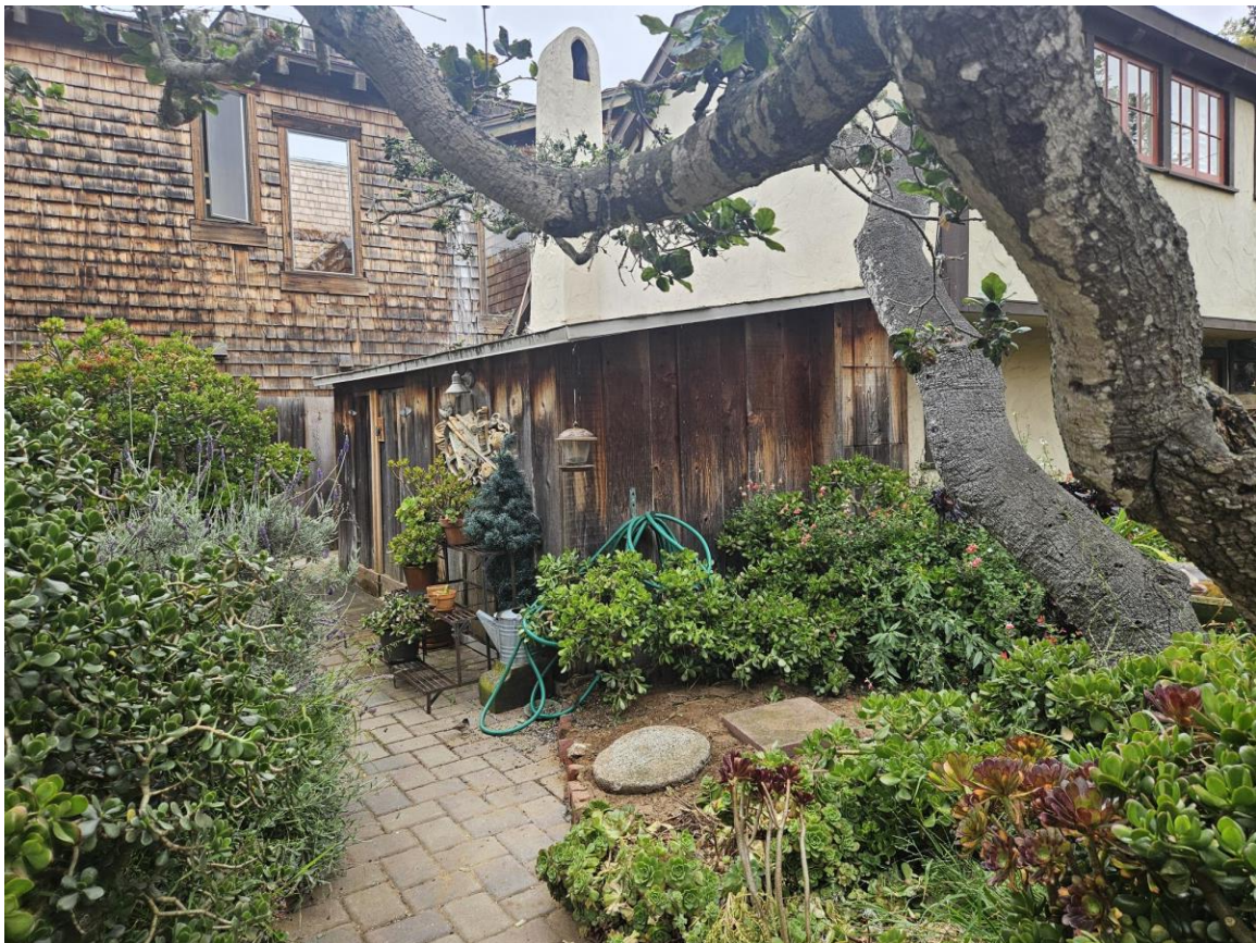
Shed behind residence.
