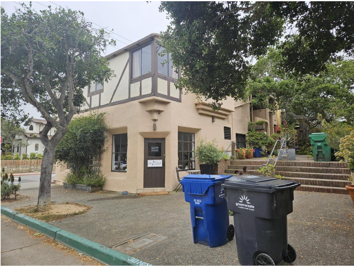
Hills Corners looking southwest.
