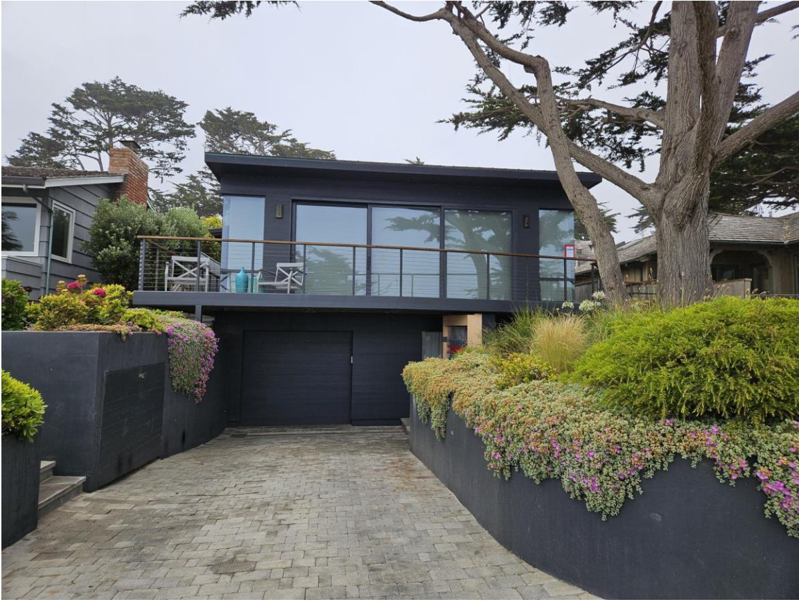
Front elevation and garage.
