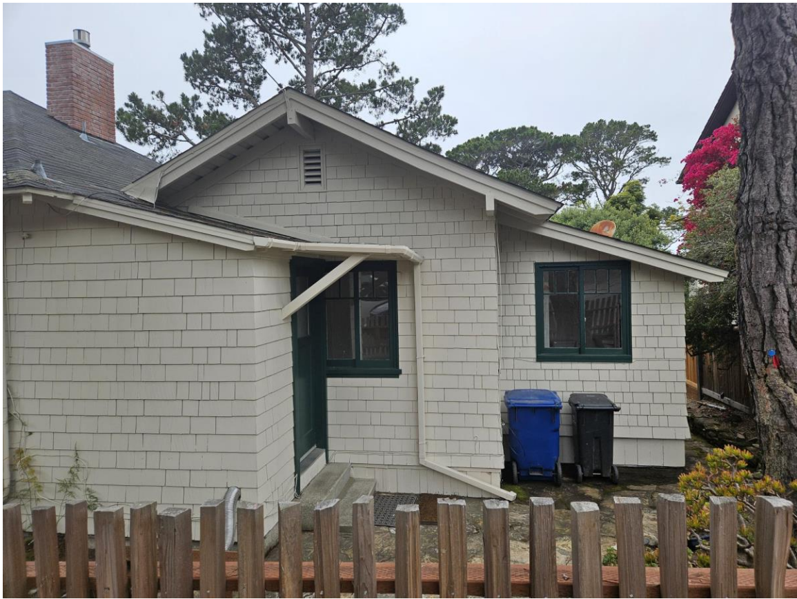
Additions at rear elevation, looking west.
