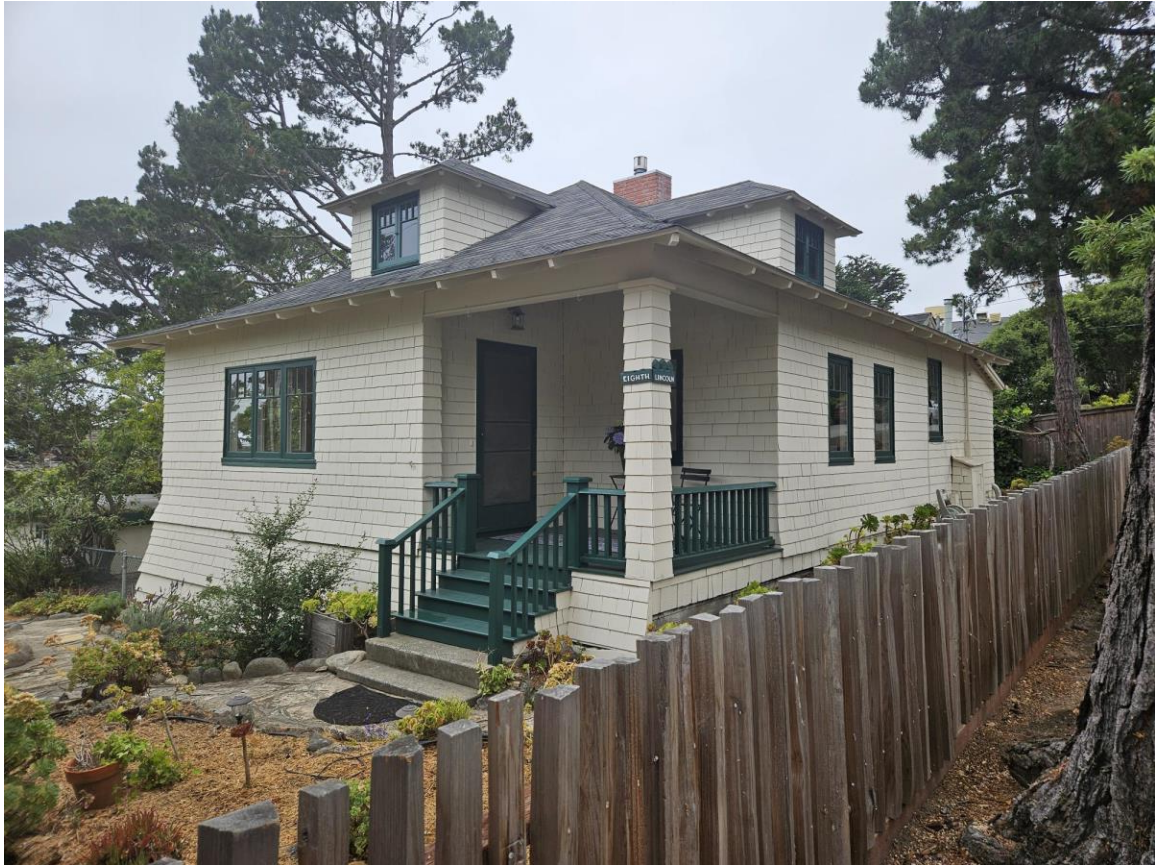
Front elevation looking northwest.
