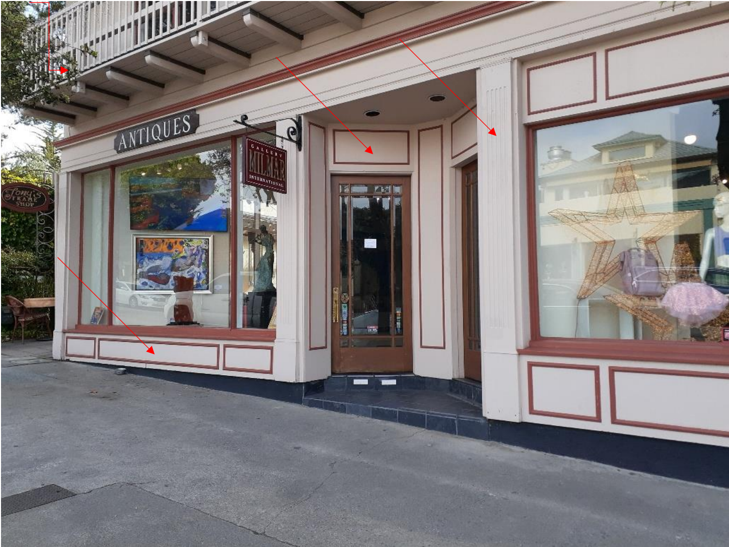
Figure 3: Arrows indicate incompatible changes to the facade
