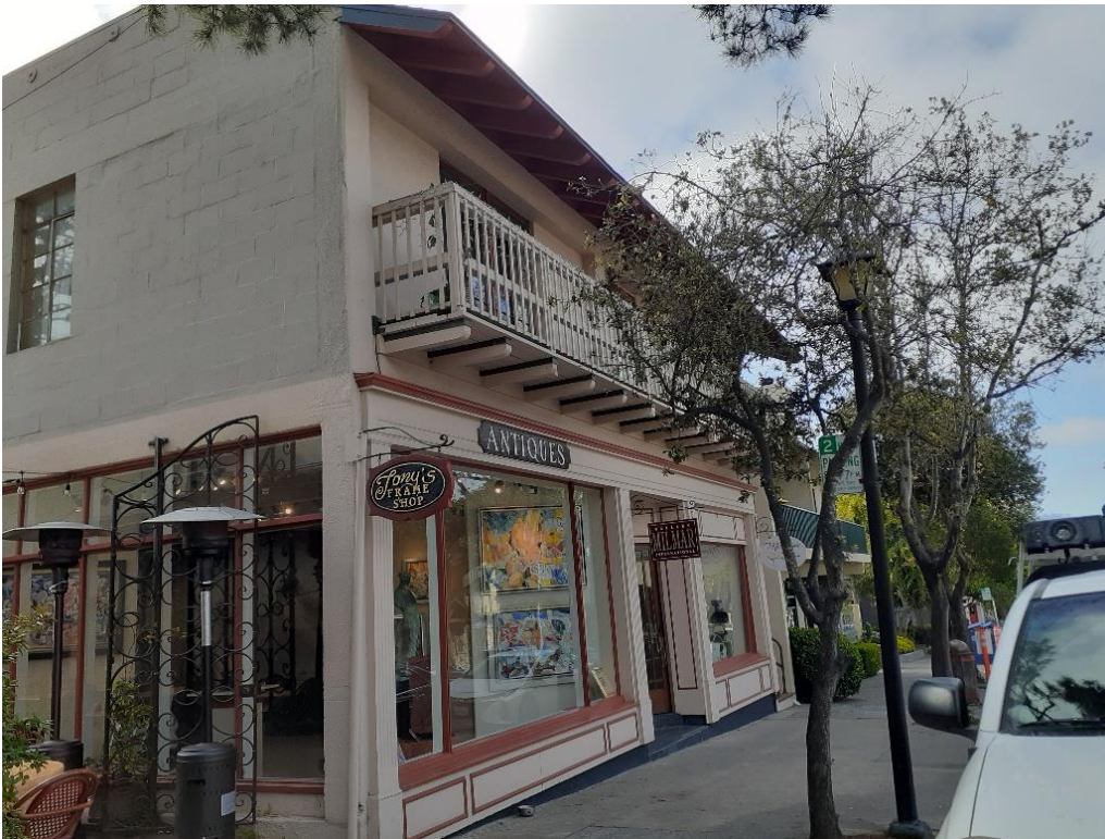
Figure 1: View of front elevation looking southeast
