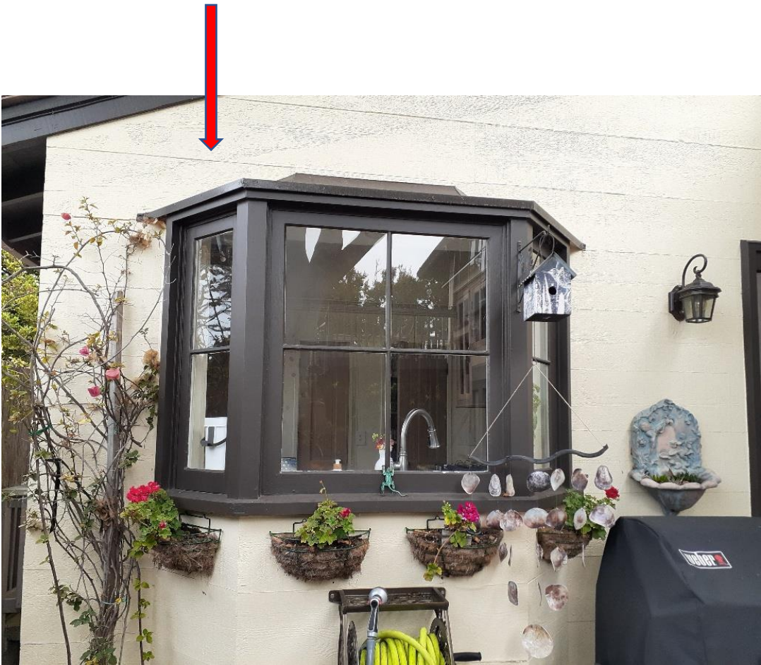
Figure 1: View of kitchen bay window & original roofline indicated by arrow
