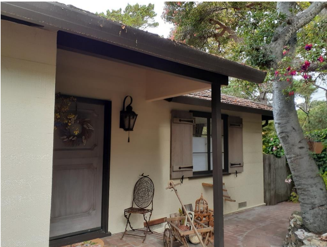
Figure 4: View of front entrance and new shutters
