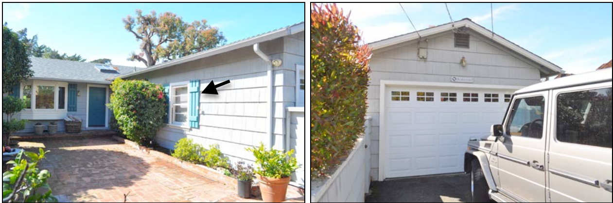
Figures 1 and 2. Left image shows the front (east) elevation. An original window exists on the south wall of the garage wing. Right image details the street-facing garage with replaced garage door.
