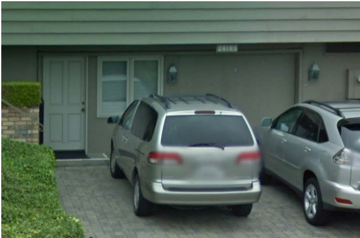
Photo 3. Front Elevation Modification/Garage Conversion at Lower Level
