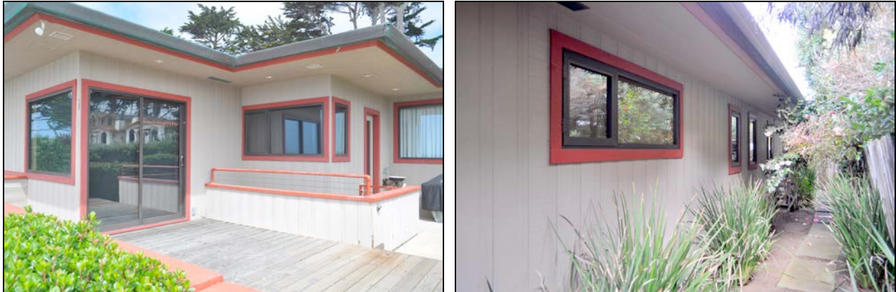
Figures 3 and 4. Left image details the side entrance on the south elevation. All original windows have been replaced with metal casements or fixed glass as part of a 2001 remodeling campaign. Right image shows the rear elevation.
