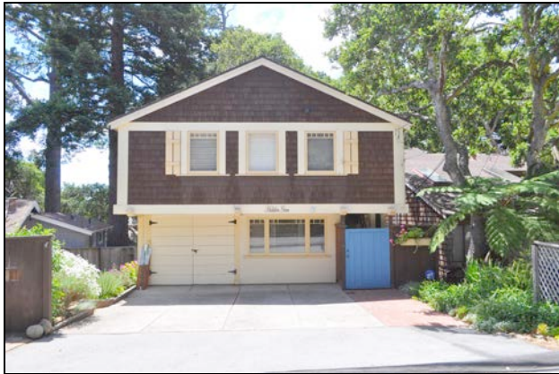
Figures 1 and 2. Left image shows the front (east) elevation facing the street. Right image details the front elevation showing the right-hand garage converted to an apartment, the stairway leading to the upper-floor entrance, the replaced upper-floor windows and the wood-shingle wall cladding.
