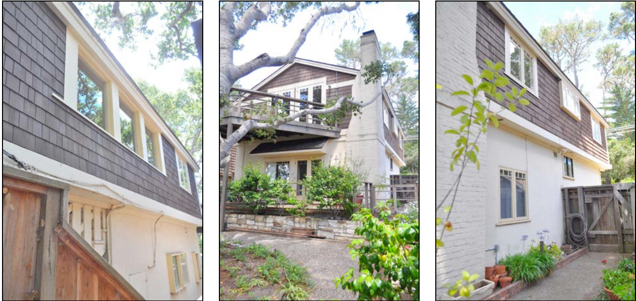
Figures 3 - 5. Left image details the right side entrance, showing infill of the upper-floor windows. Center image shows the rear elevation, with painted southwest corner chimney and replaced second floor doors. Right image shows the left side elevation looking toward the street.
