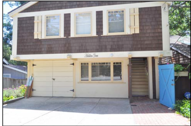
Figures 1 and 2. Left image shows the front (east) elevation facing the street. Right image details the front elevation showing the right-hand garage converted to an apartment, the stairway leading to the upper-floor entrance, the replaced upper-floor windows and the wood-shingle wall cladding.
