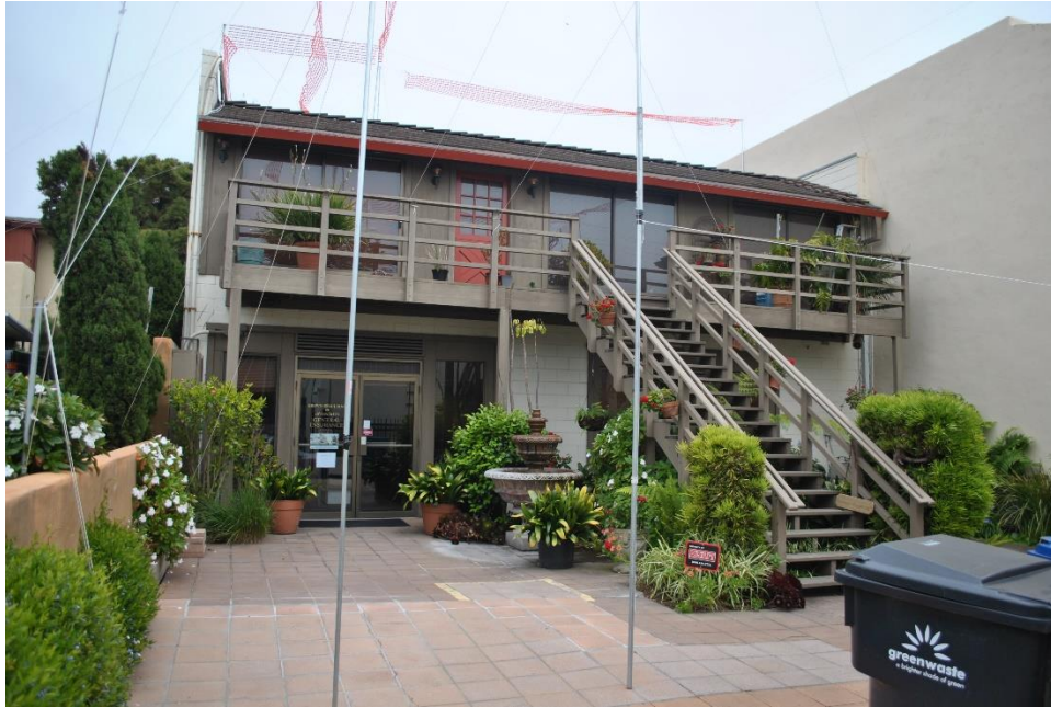
Figure 2: West Elevation. Concrete block building constructed in 1970.
