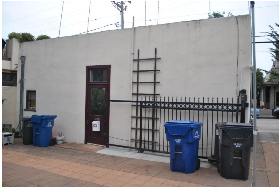
Figure 3: East elevation. Rear of 1946 office and store building.
