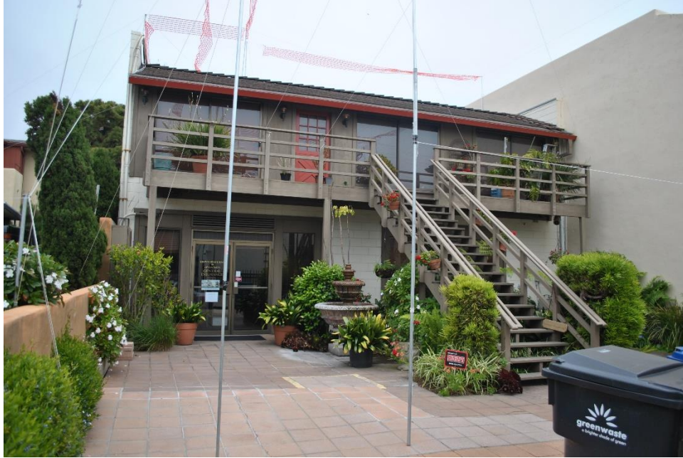
Figure 2: West Elevation. Concrete block building constructed in 1970.
