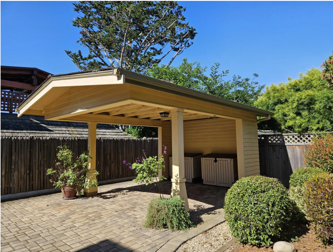
Figure 5: View of carport looking southwest.
