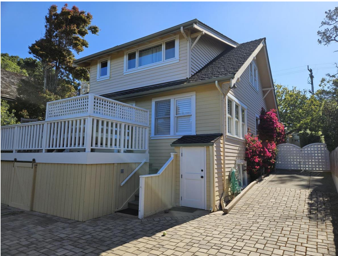
Figure 4: View of rear and south elevations.
