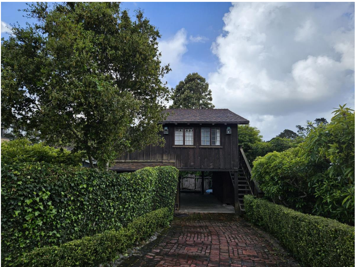
View of 1972 addition over the carport and exterior stairs.
