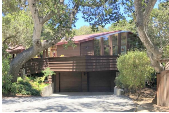
Mark Mills' Walker Spec House (1951) at Rio Road and Thirteenth Avenue.
