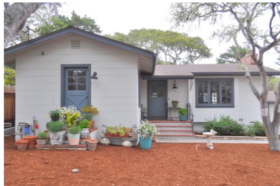
Alta R. Jensen House (1947) by Edwin Lewis Snyder at Torres Street 5 NE of Eighth Avenue.
