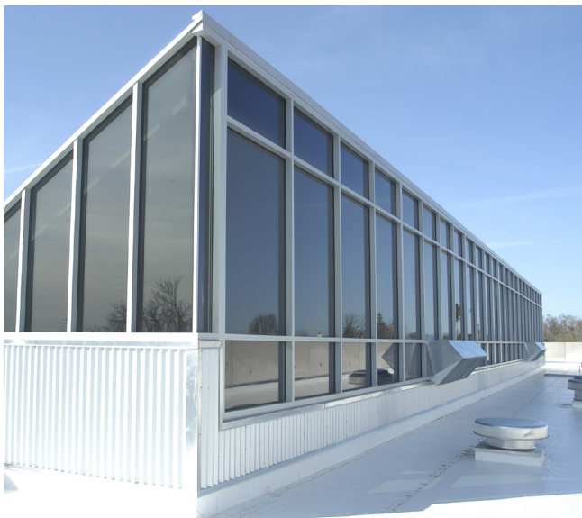
SKYLIGHT ON LEED CERTIFIED POLICE HEADQUARTERS, WOODLAND, CA
