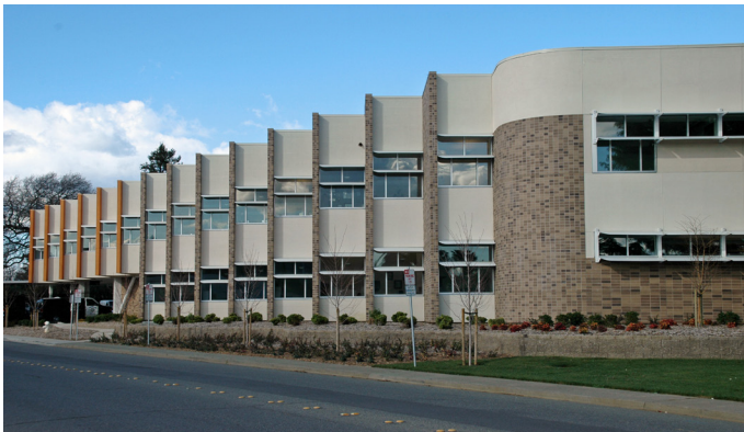
STAGGERED EXTERIOR OF THE VACAVILLE POLICE HEADQUARTERS, USE SHADED SOUTH FACING WINDOWS TO IMPROVE INTERIOR DAYLIGHT WHILE MINIMIZING HEAT GAIN
