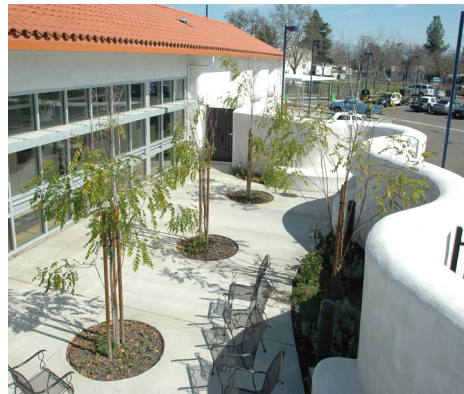
STRAWBALE WALL AND COURTYARD AT THE VISALIA POLICE SUBSTATION
