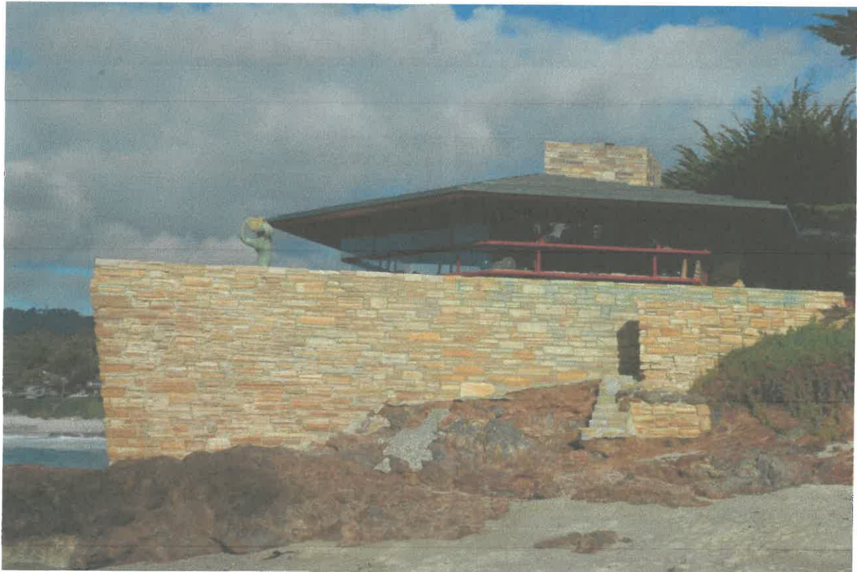
Pattern of stone veneer on south face.
