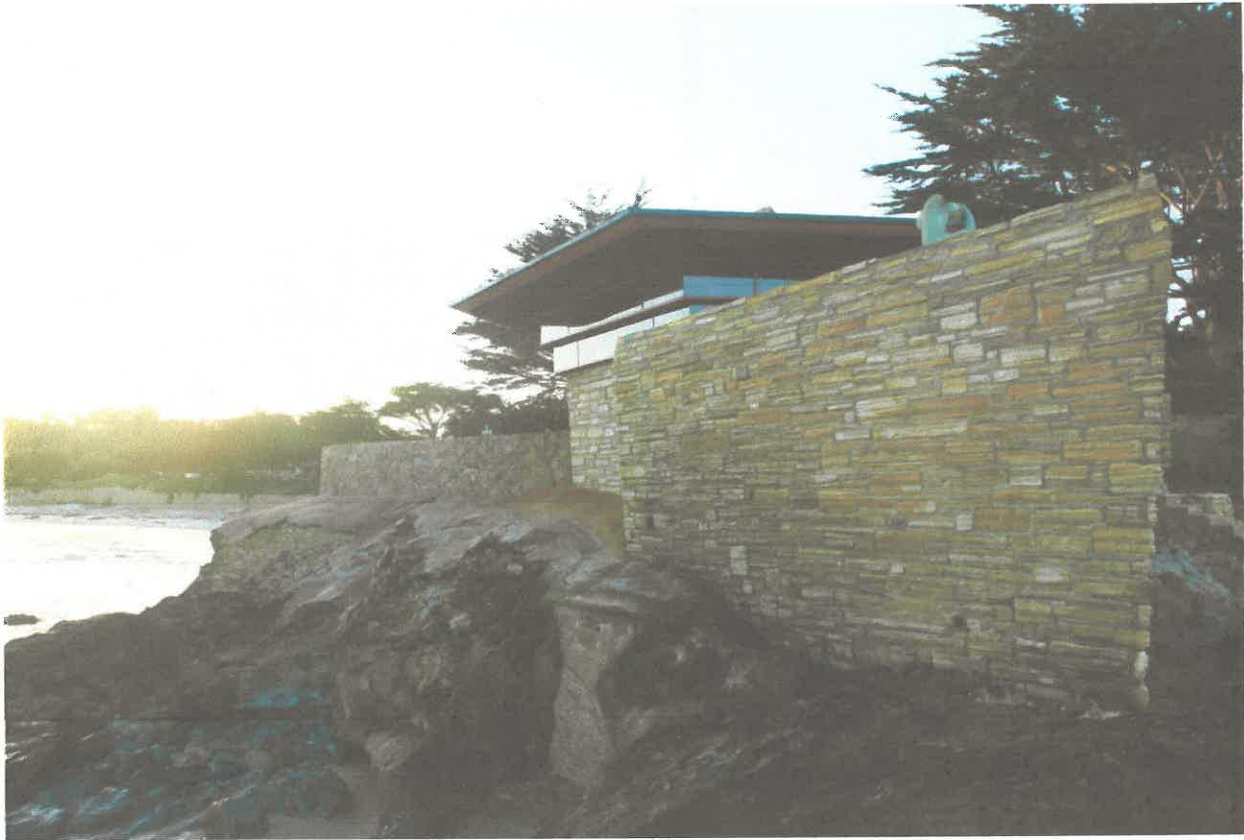
Pattern of stone veneer on northwest face.
