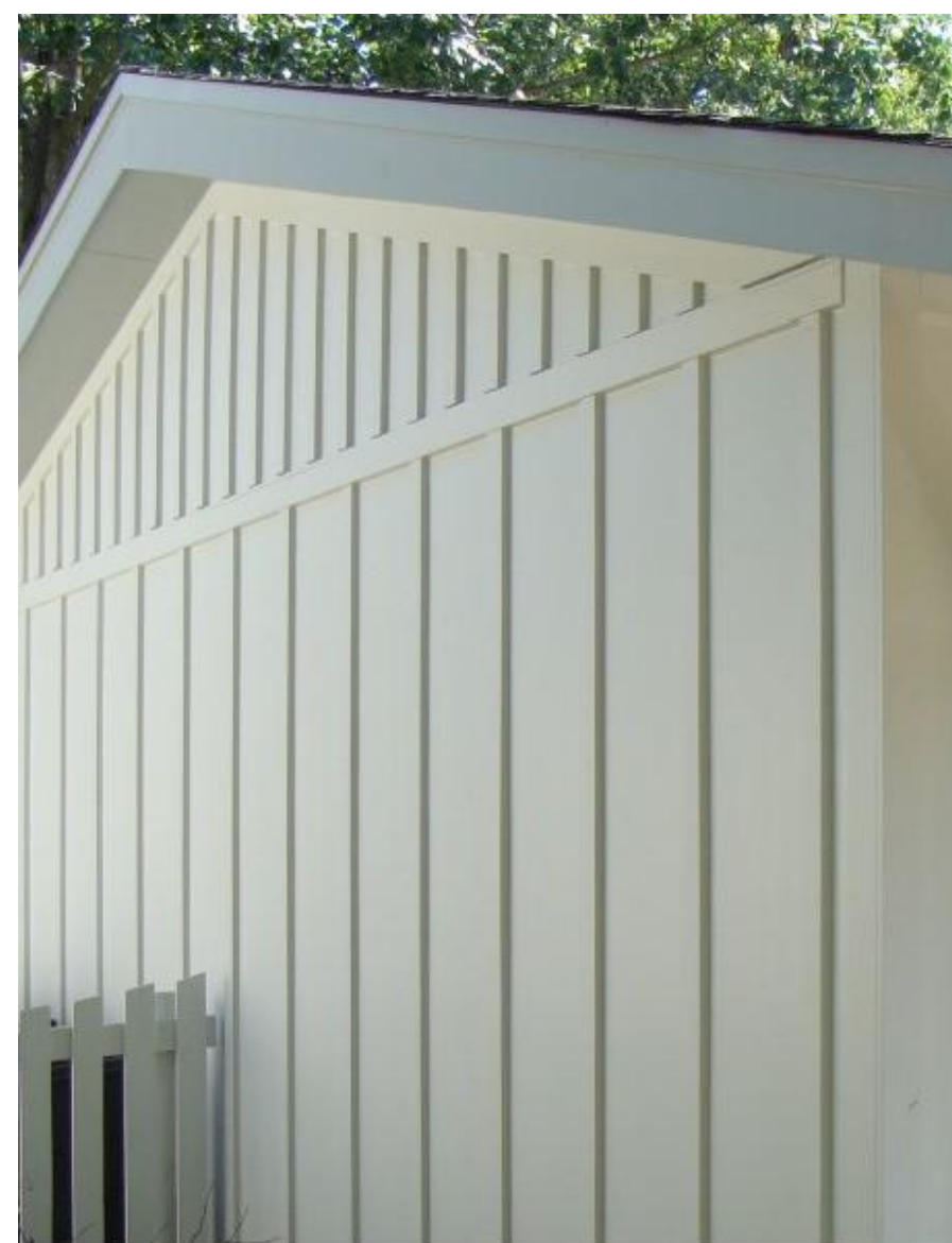
4 PAINTED WOOD. BOARD & BATTEN SIDING COLOR: WHITE
