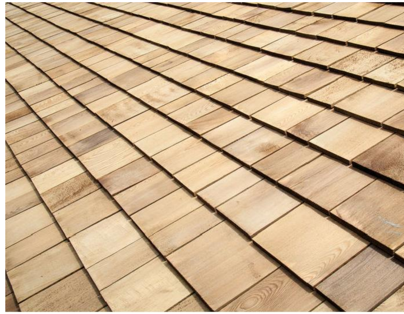
1 CLASS 'A' WOOD CEDAR SHAKE ROOF
