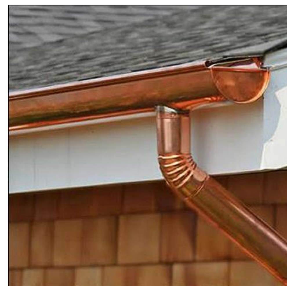
7 COPPER GUTTERS AND DOWNSPOUTS
