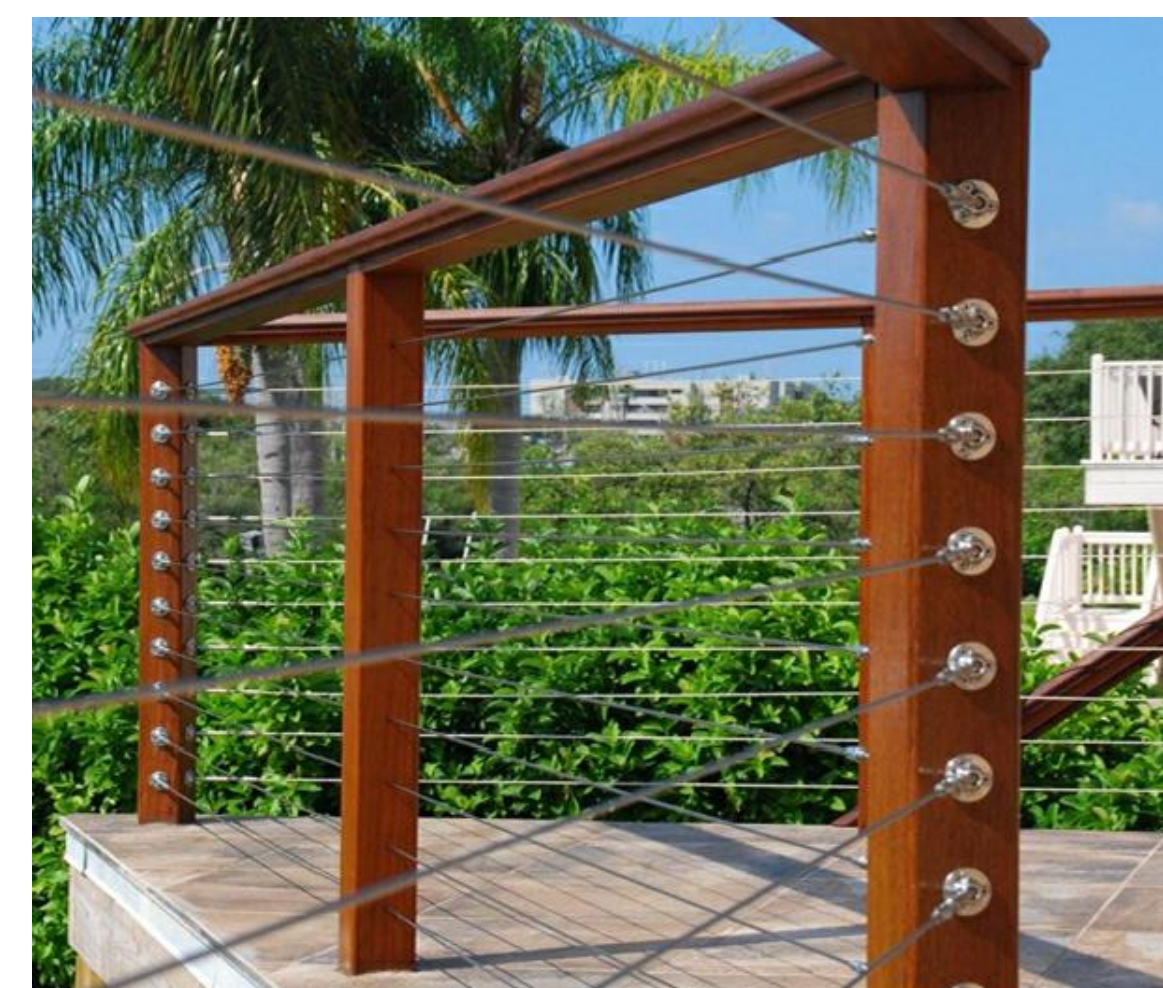
8 CABLE RAILING W/ REDWOOD TOP RAIL
