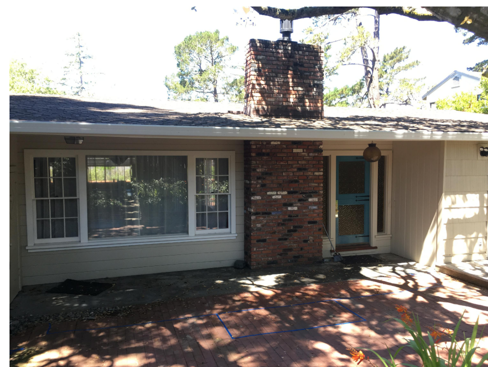
FRONT ELEVATION LOOKING WEST
