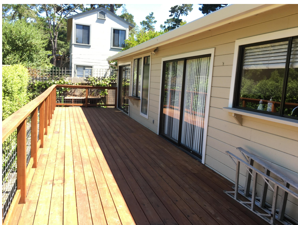
EXISTING DECK LOOKING NORTH
