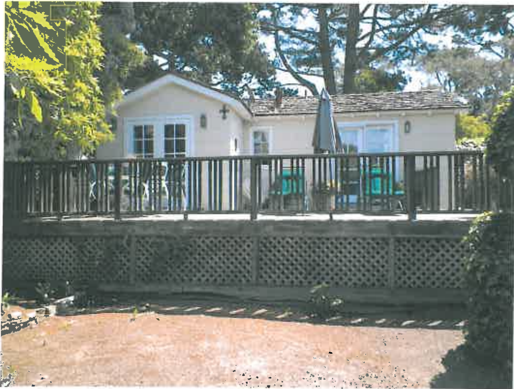
Project Site – Rear of residence facing east
