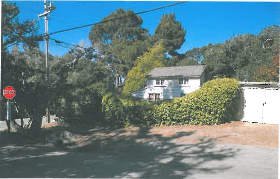
Project site from 11th Ave looking at the attic proposed for a 2 nd story addition
