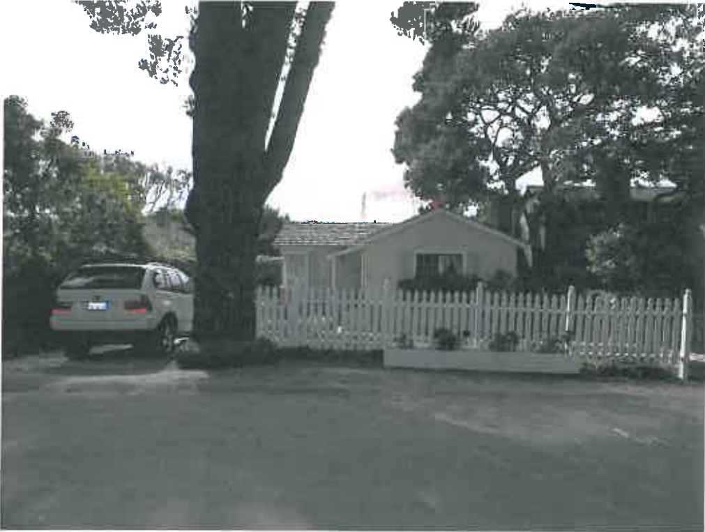
Project site – Facing west on Camino Real
