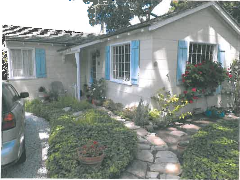
Project Site – Front of residence facing west
