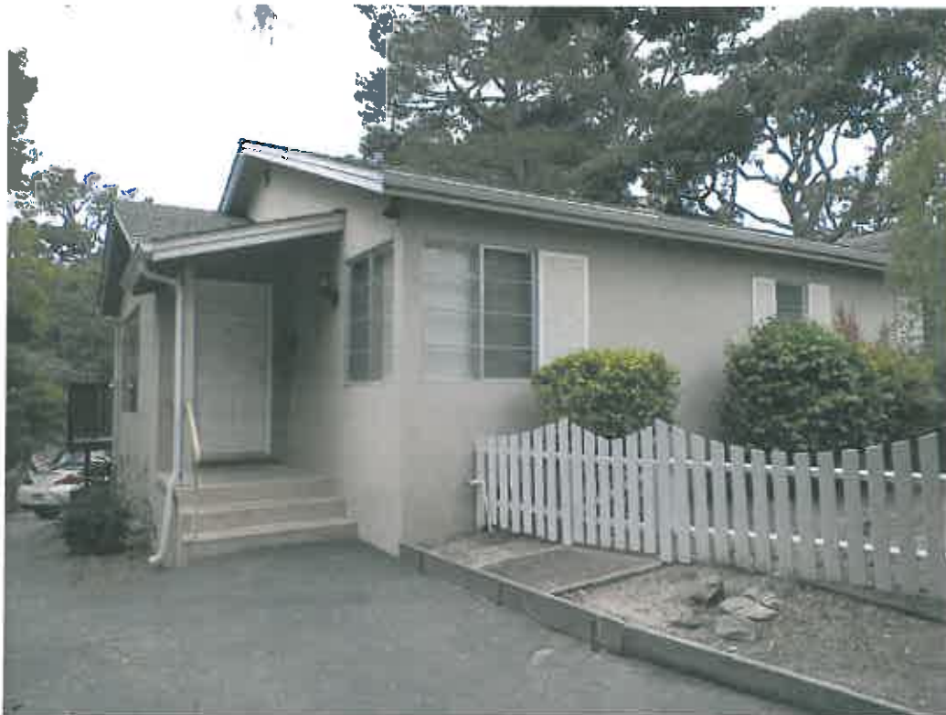
Project site – Front of residence facing west
