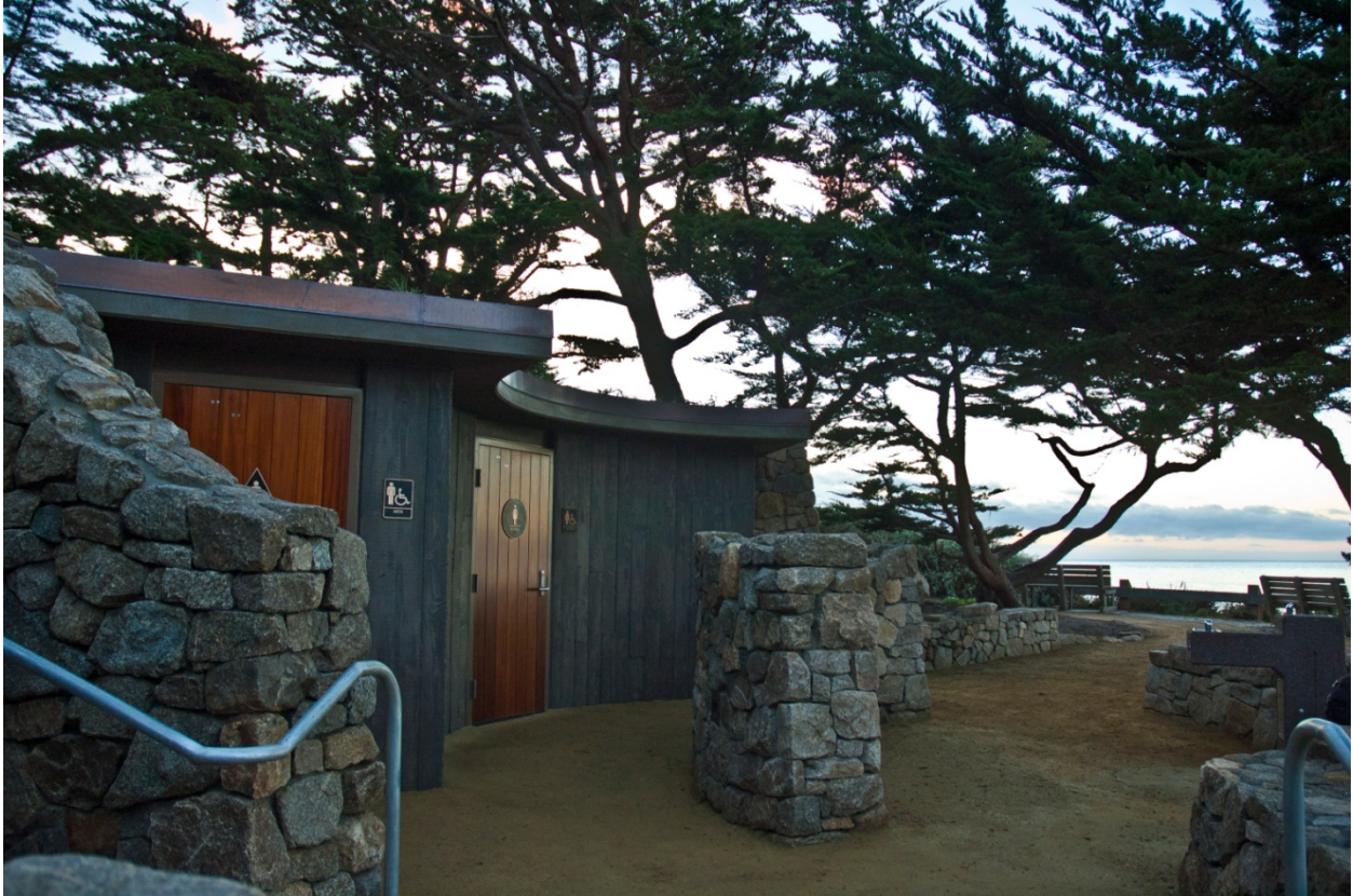
Restroom Facility – Facing south
