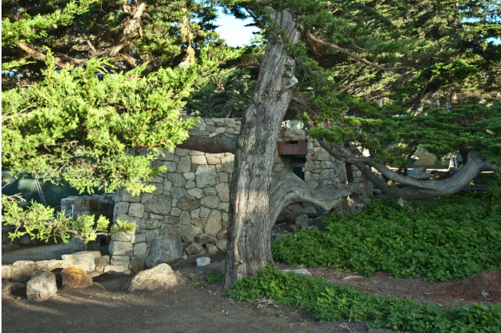
Back of Restroom – Facing north
