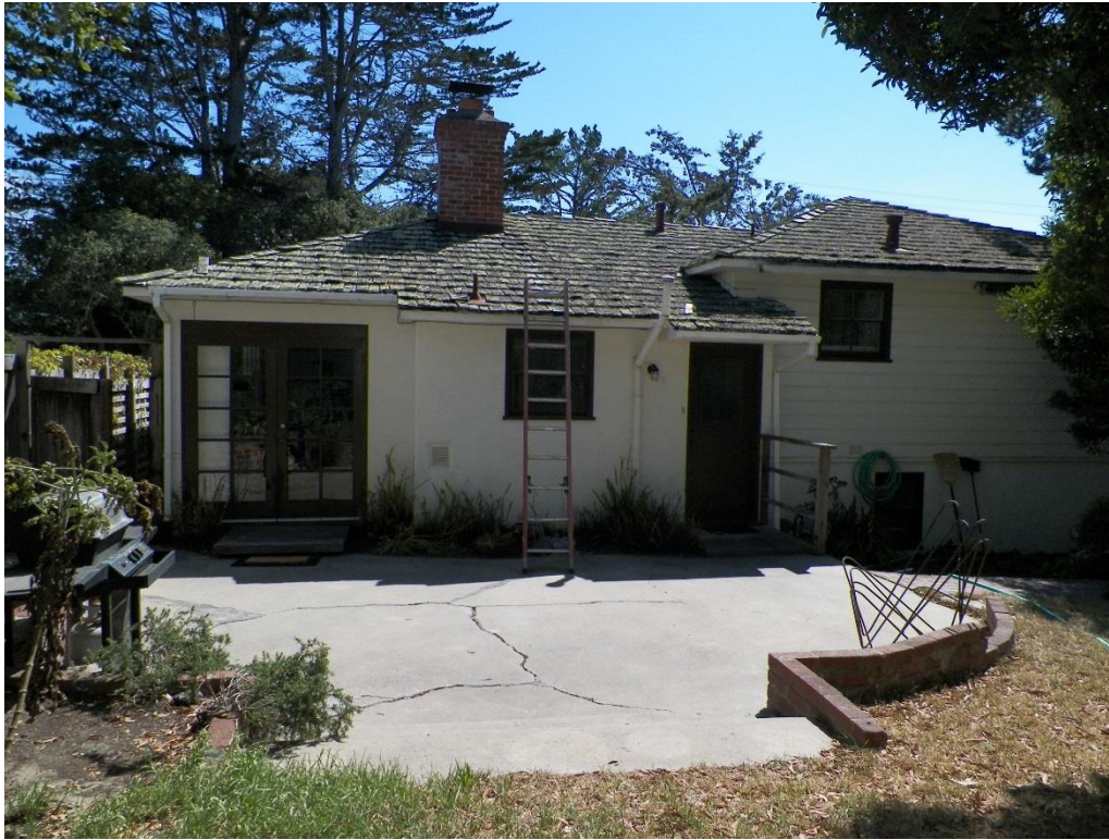
Project Site – Rear (North) Elevation
