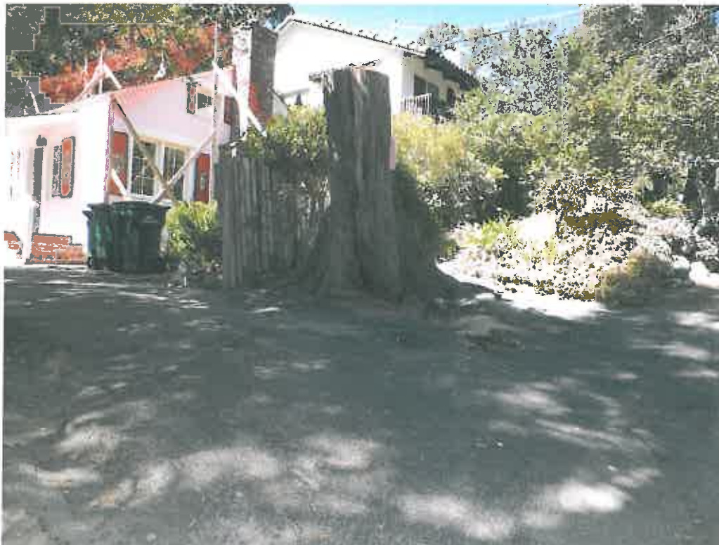
Project site – Facing northwest on Monte Verde Street showing excess pavement in ROW
