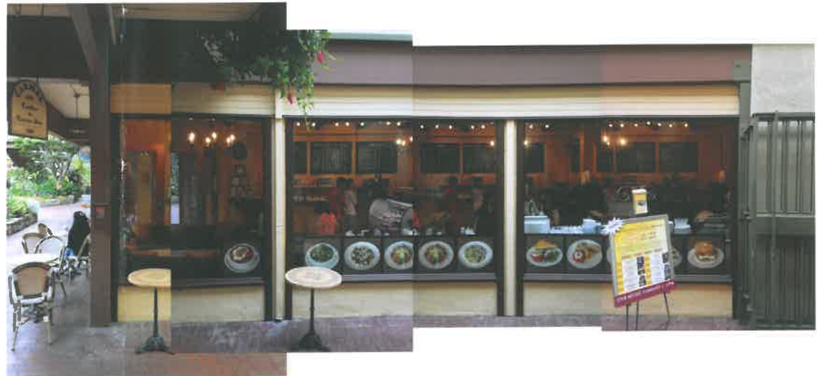
VIEW OF NORTH STOREFRONT
