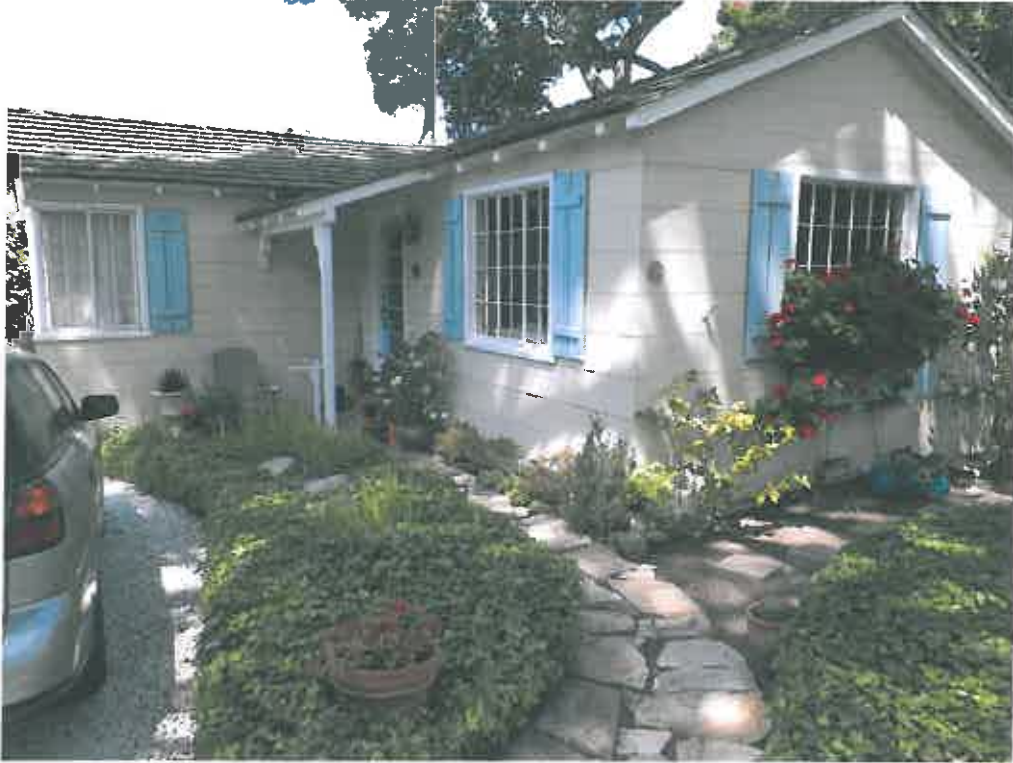
Project Site – Front of residence facing west
