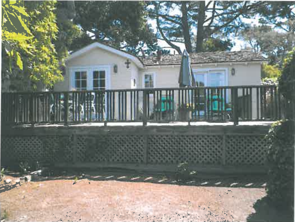
Project Site – Rear of residence facing east
