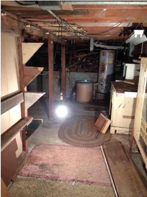
Crawlspace below residence
