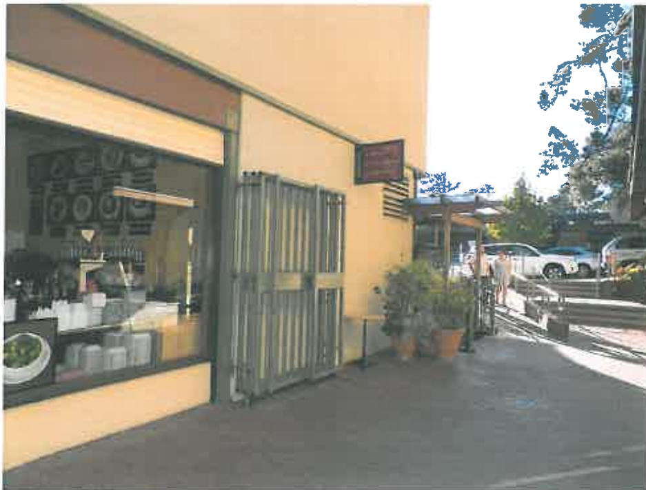
Project Site –North Elevation of Carmel Coffee, looking towards Mission Street
