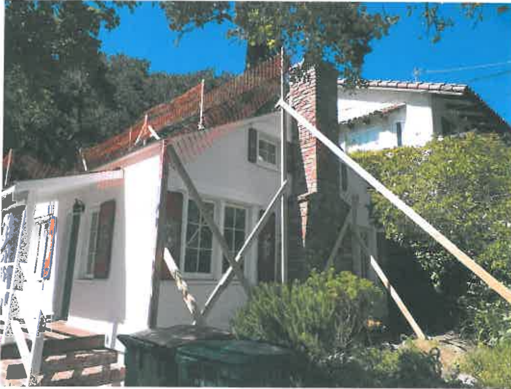
Photo taken from project site – Facing northwest
