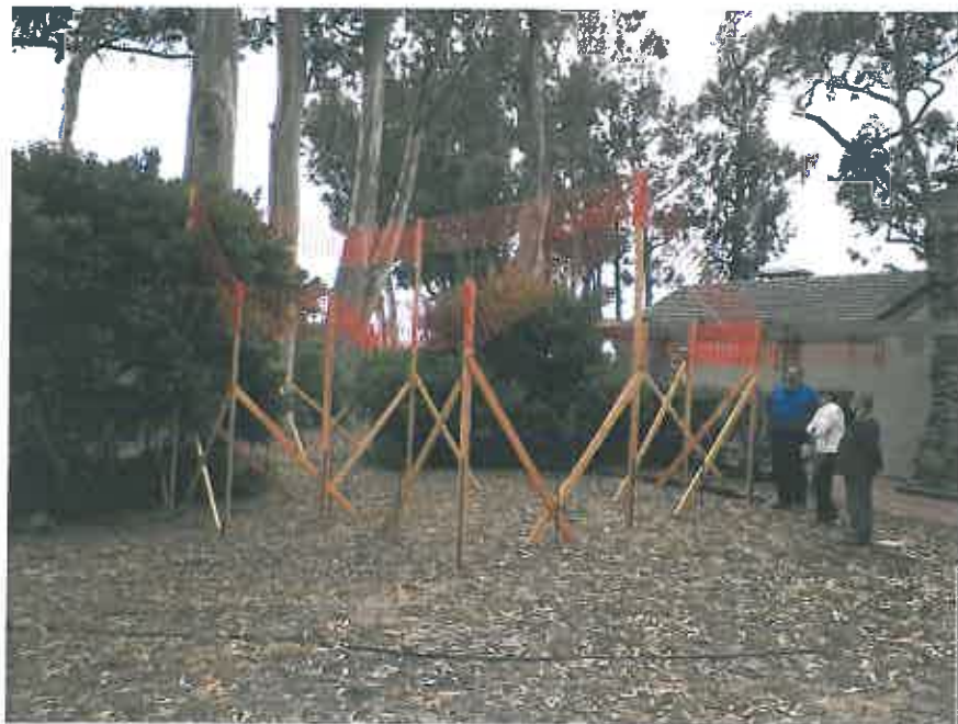
Project Site – Facing north area of addition (original story-poles)
