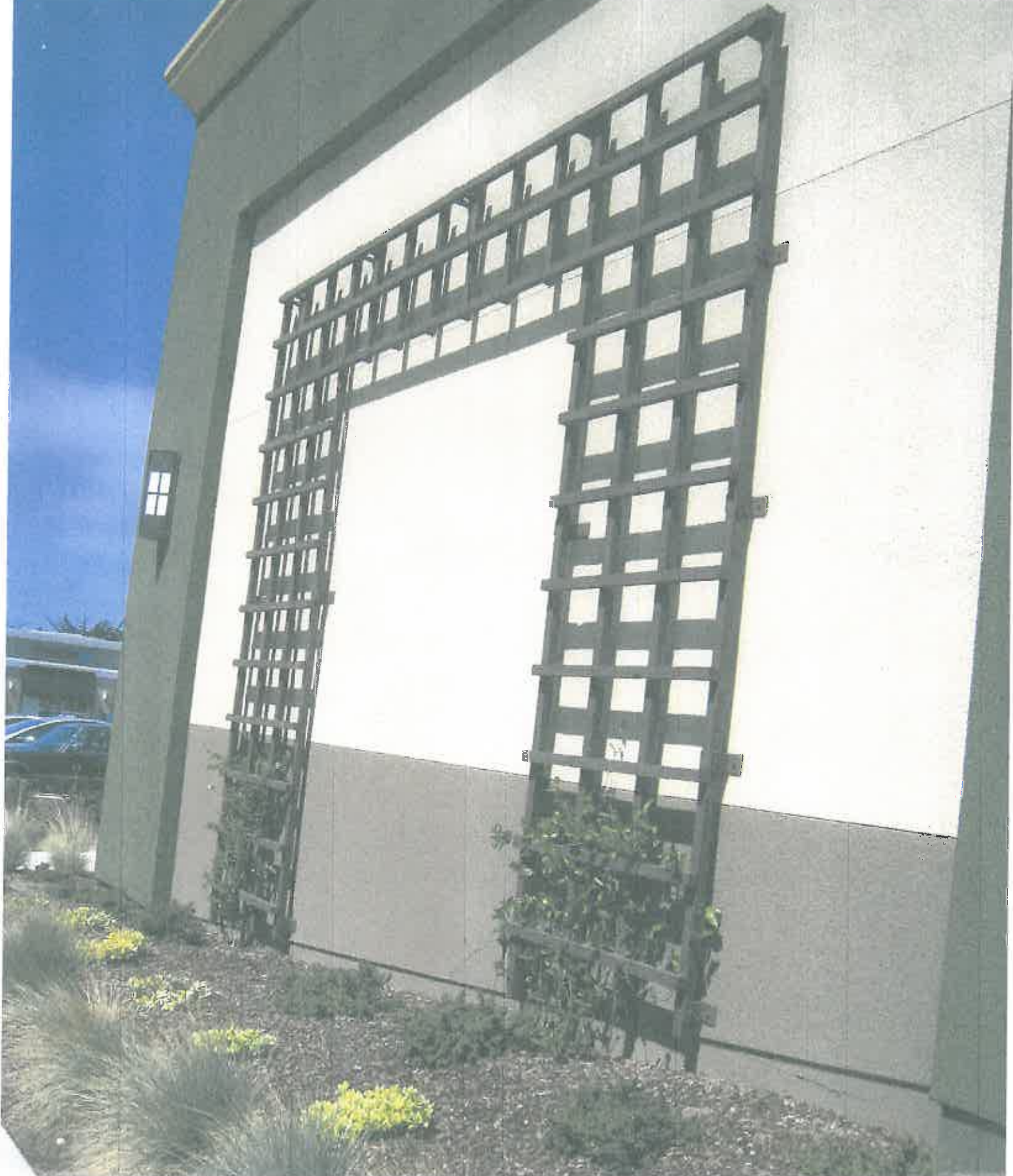
ALTERNATE CONSTRUCTION OF LIVING WALL GORDON
