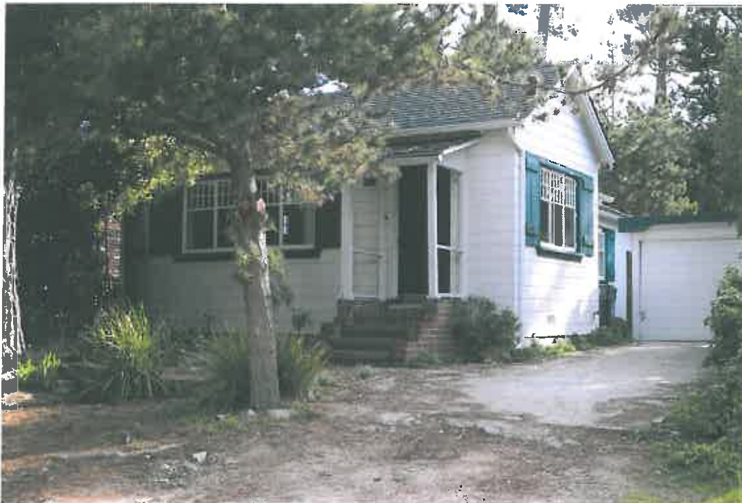
Front of residence along Torres St.
