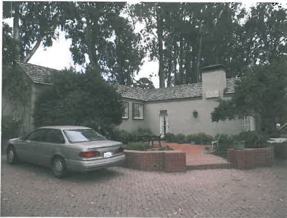
Project site - Rear of residence facing southeast
