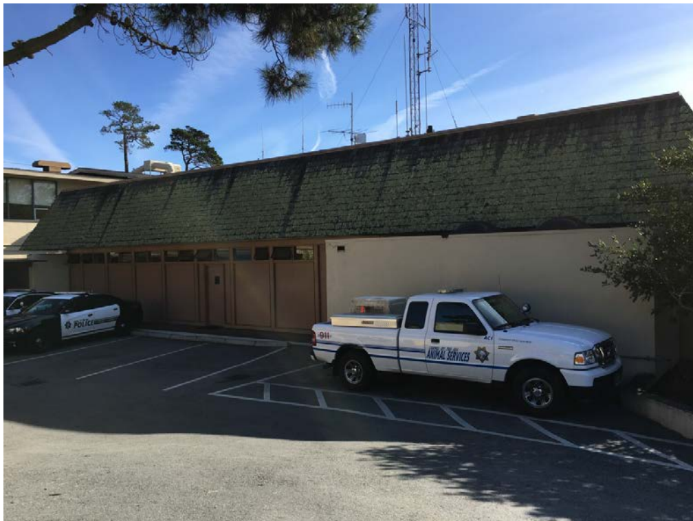
Photo 3. PD north elevation
