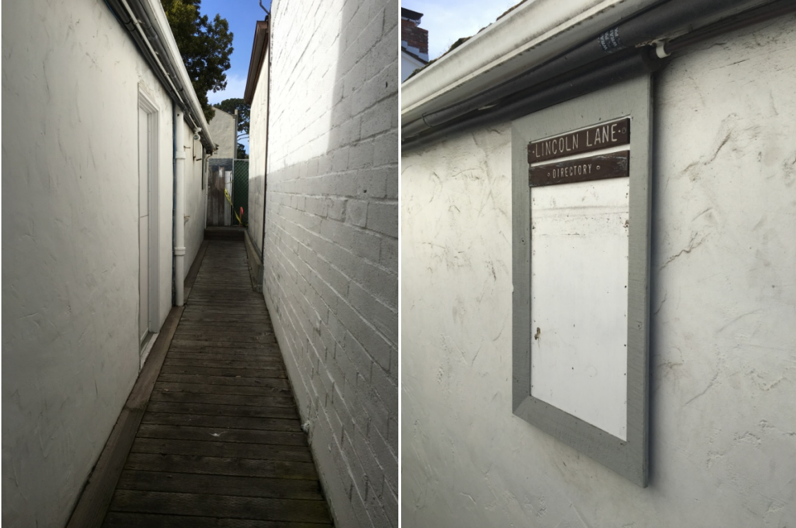
Existing Intra-Block Walkway at the rear of Lincoln Lane
