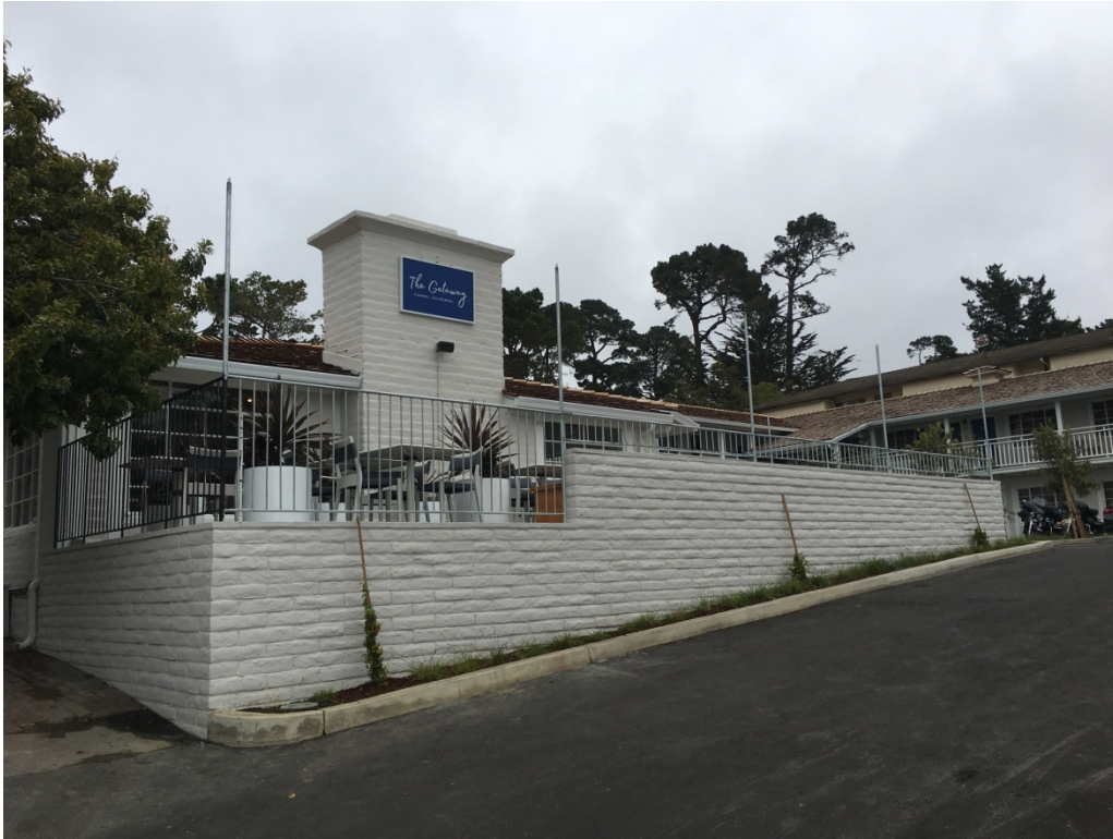
Photo 1. New Outdoor Patio @ The Getaway (formerly The Village Inn)
