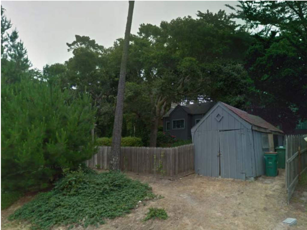
Photo 1. Existing Single Car Detached Garage (Dolores Street)
