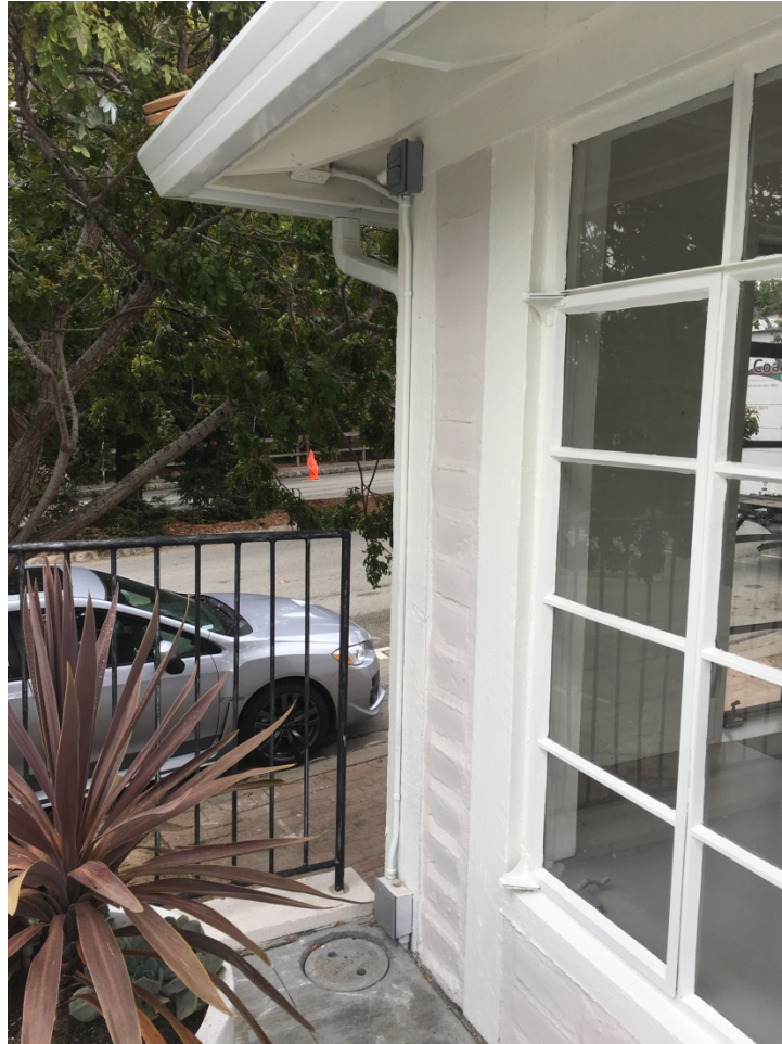
Photo 3. Hard-wired Exterior Electrical Outlets
