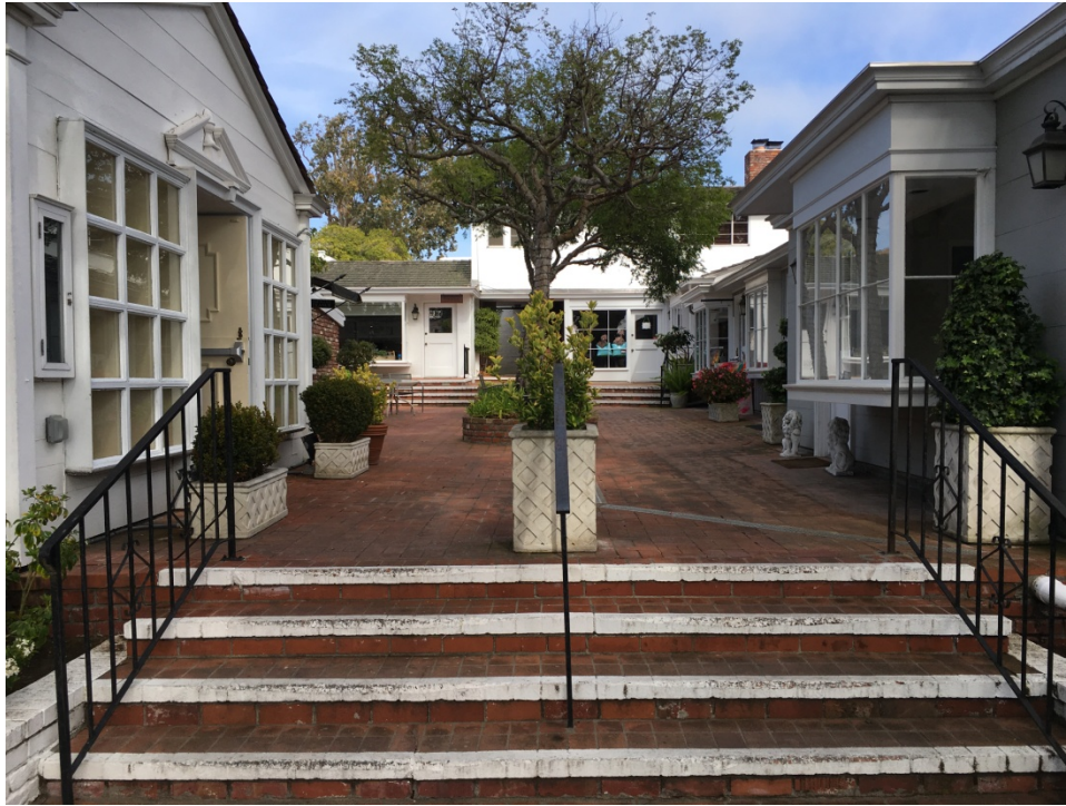
Existing courtyard entry from Lincoln Avenue
