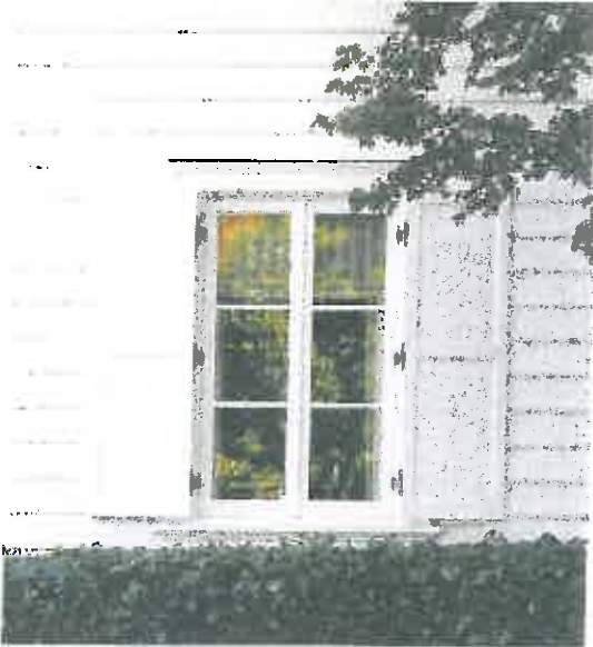
Painted wood casement windows with divided lites and painted wood trim
