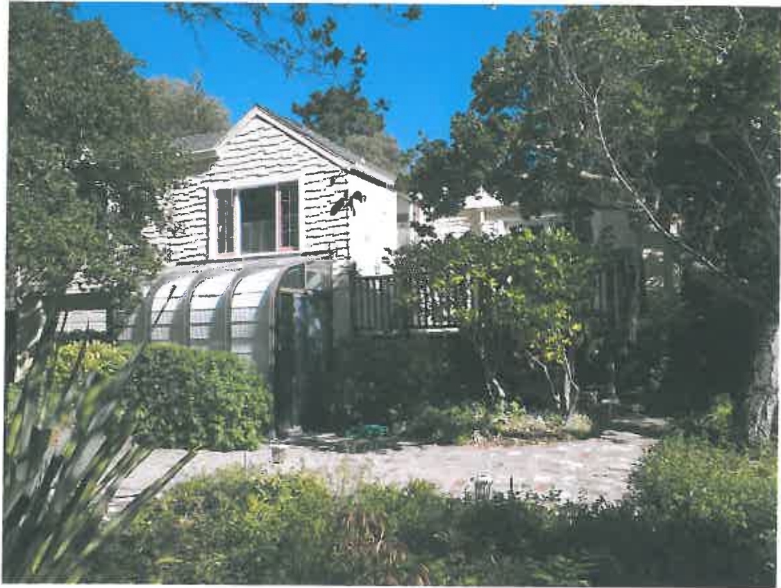
Rear of the property facing east
